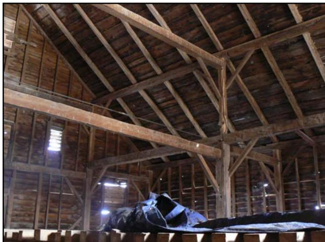
Photo 9. Interior of the Jacob Post barn, showing bents with later vertical extensions (Ned Pratt).
