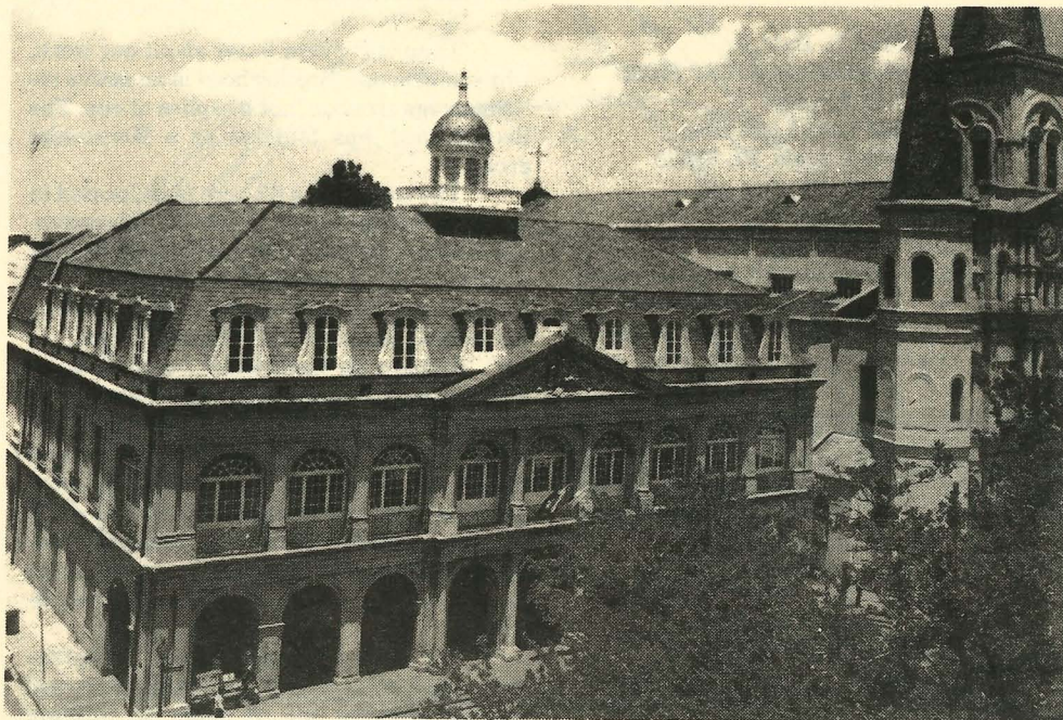
The Cabildo, Jackson Square, New Orleans, Louisiana, as it appeared before the 1988 fire. Photo courtesy of Koch & Wilson Architects, New Orleans.
