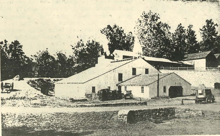
Hopewell Furnace National Historic Site, Elverson, Pennsylvania.
