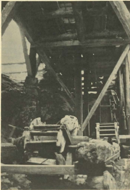
3.) Sawmill, Telemark, Norway. From under the sawmill we see the small water wheel which returns the log-carriage, and behind that the flutter wheel which drives the blade.
