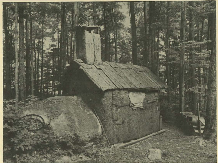
Jack Leadley's Bark Shanty . The north side of the shanty is built against the flatside of a granite boulder. Inside, the stone wall serves as the back for the open firewhich burns in a shallow pit at its base. A rawhide deer skin serves as a window. Jack prefers sleeping here than to sleeping in the house (Photo by P. Sinclair)
