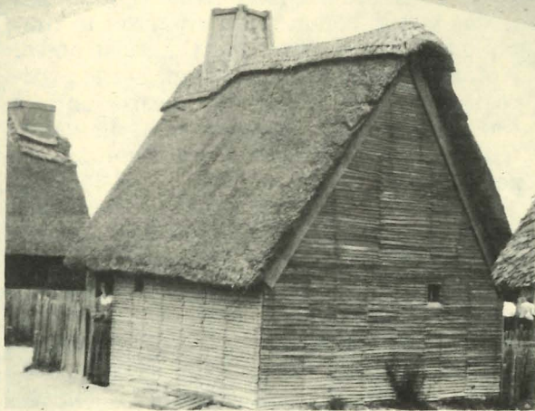
(LEFT) Isaac Allerton House, Plymouth Plantation 1976. The house is finished with riven clapboard and roofed with reed thatch.. photo by Don McTernan
