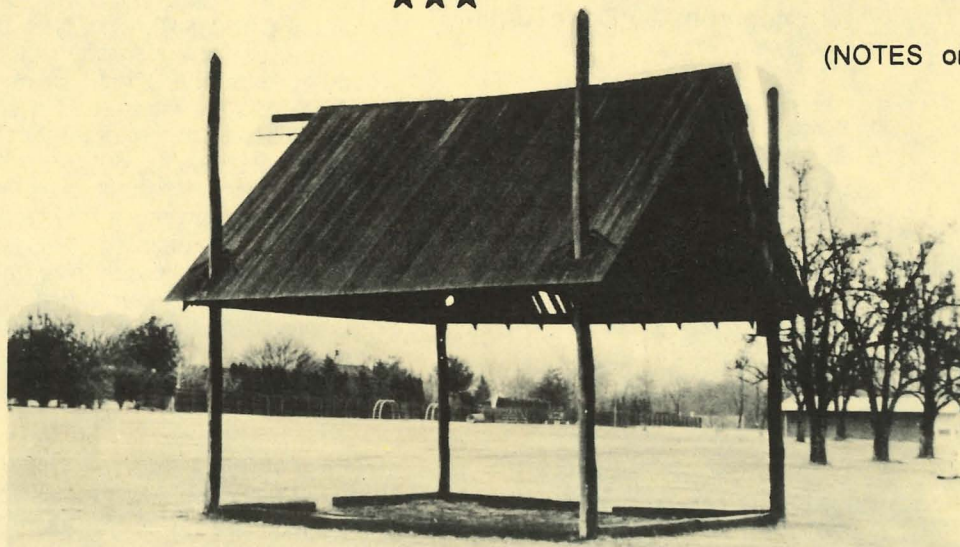
Hay Barrack in Hackettstown, New Jersey, 1977 . The gable roof became popular on later barracks, which were covered with thin vertical boards. Some had hay tracks like this one to facilitate unloading loose hay from a wagon.
