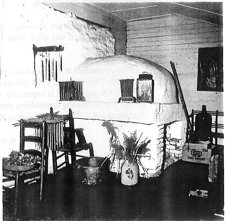
Dome of bake oven within leanto on east end of kitchen wing
