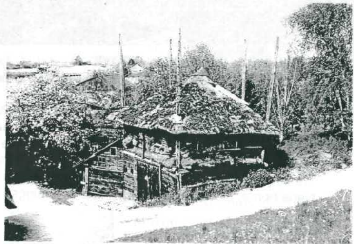
5-Pole Barrack ( steltenberg ) bellow the dike along the river Waal
