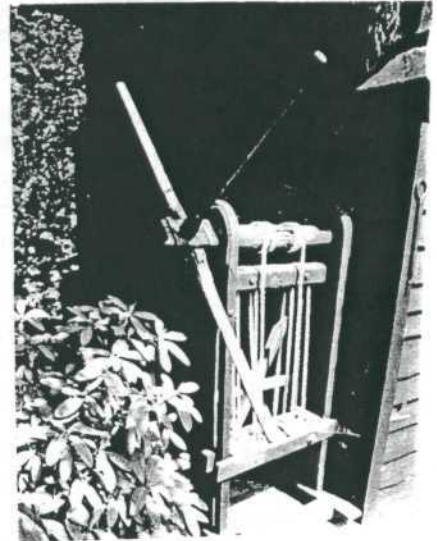
Capstan ( heeft ) used to raise roofs of large barracks. Martin Jansen Collection
