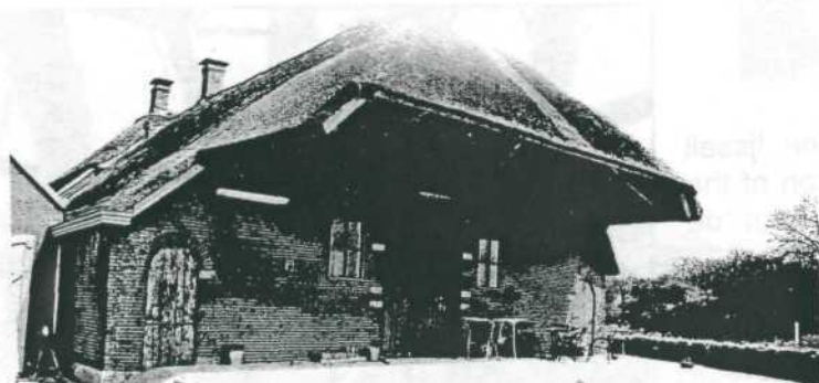
Guelderland House Barn with overhanging wolf-roof ( wolfdak )
