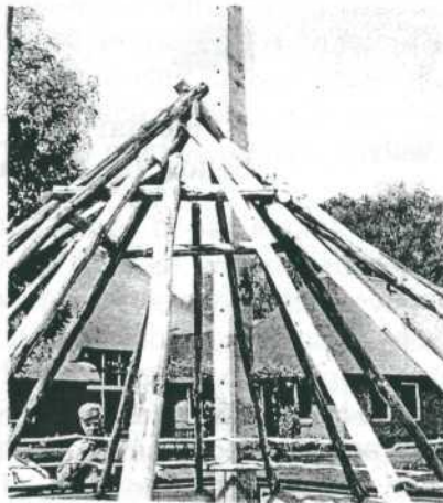
Four-Pole Hay Barrack at Hoonhorst being built by Willem Ruhoff
