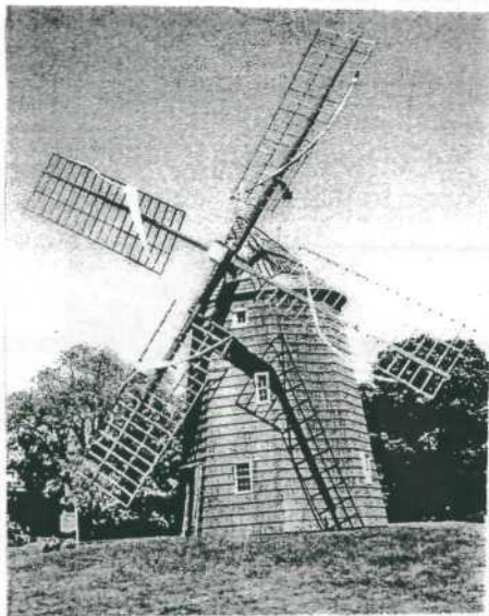
Hook Windmill, East Hampton, Long Island, NY Built 1806 to replace post-mill built in 1738. Central post of earlier mill re-used.
