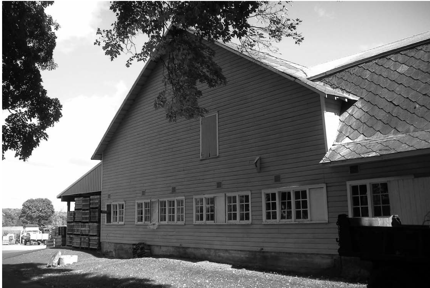
Exterior shot of the Schoonmaker eight-bay barn in Rochester Township, Ulster County. Additions at either side of the barn plus the windows at bottom of end wall are modern.
