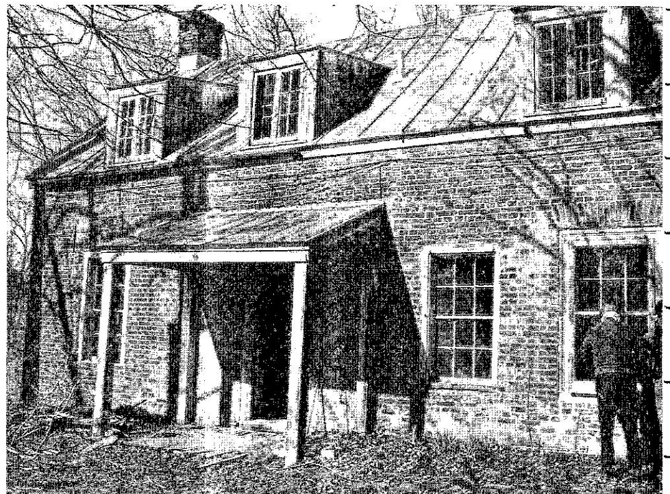
South front of the Skinkle house.
