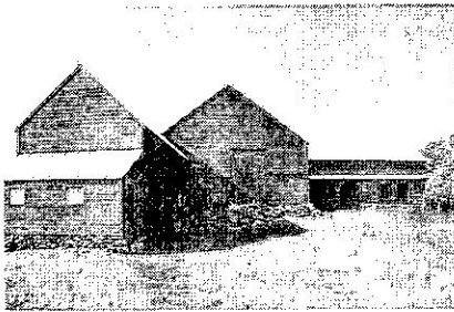
Adriance barn complex – South view of the main barn
