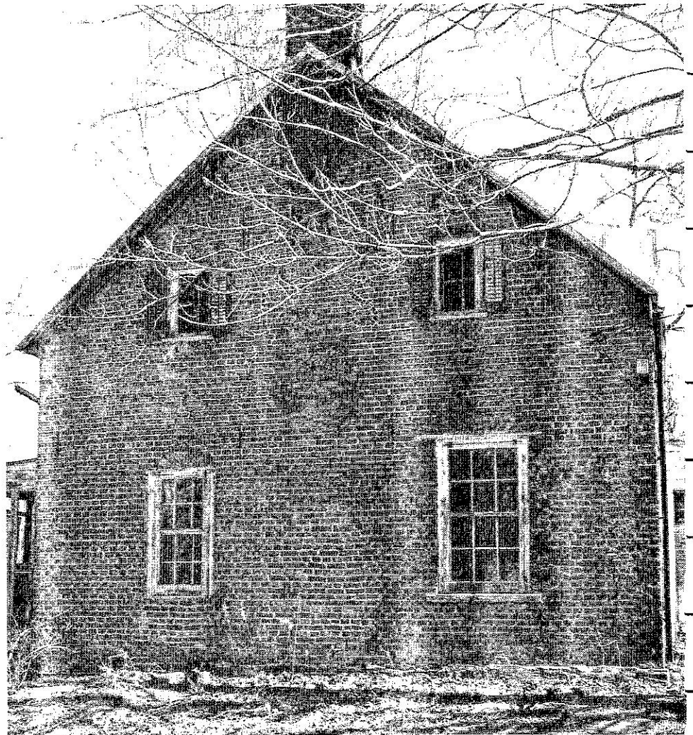
West end wall of the Skinkle house.
