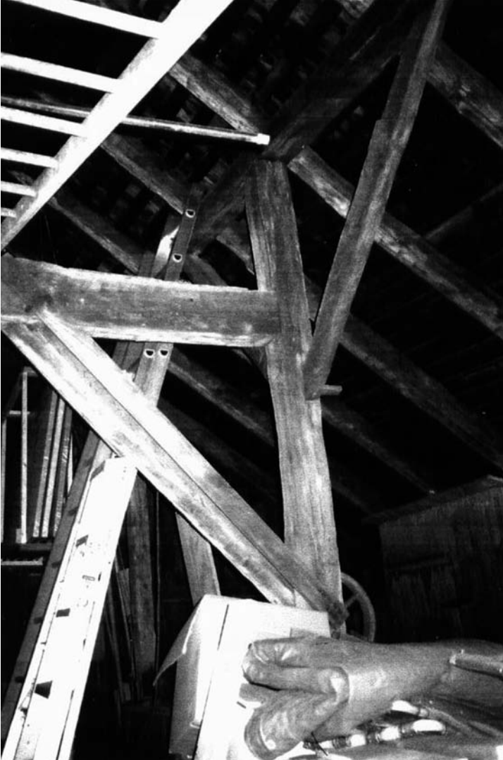
Post and anchor beam inside the Jericho Barn.
