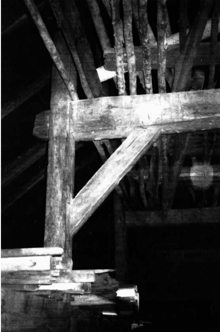
Post and anchor beam inside the Van Deusen Barn.
