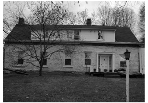
BELOW: The Mula house, Ulster, is much improved with the removal of a large enclosed porch from its facade.
