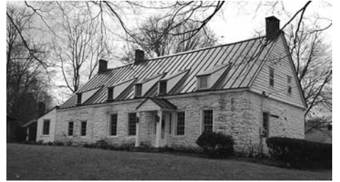
ABOVE: Glen and Jane Vinning put a fine new roof on the Osterhoudt House in Ulster.
