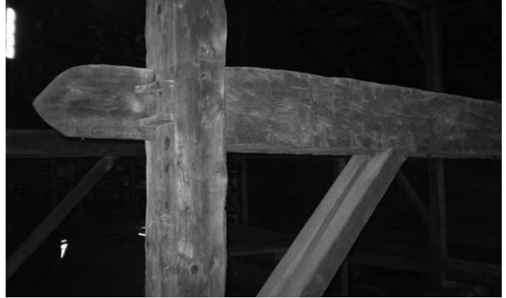
ABOVE: Middle bent is seen at its north end with anchor-beam to post juncture with prominent 19 inch long tenon extension with double wedges. Anchor-beam is oak while the post is pine.
