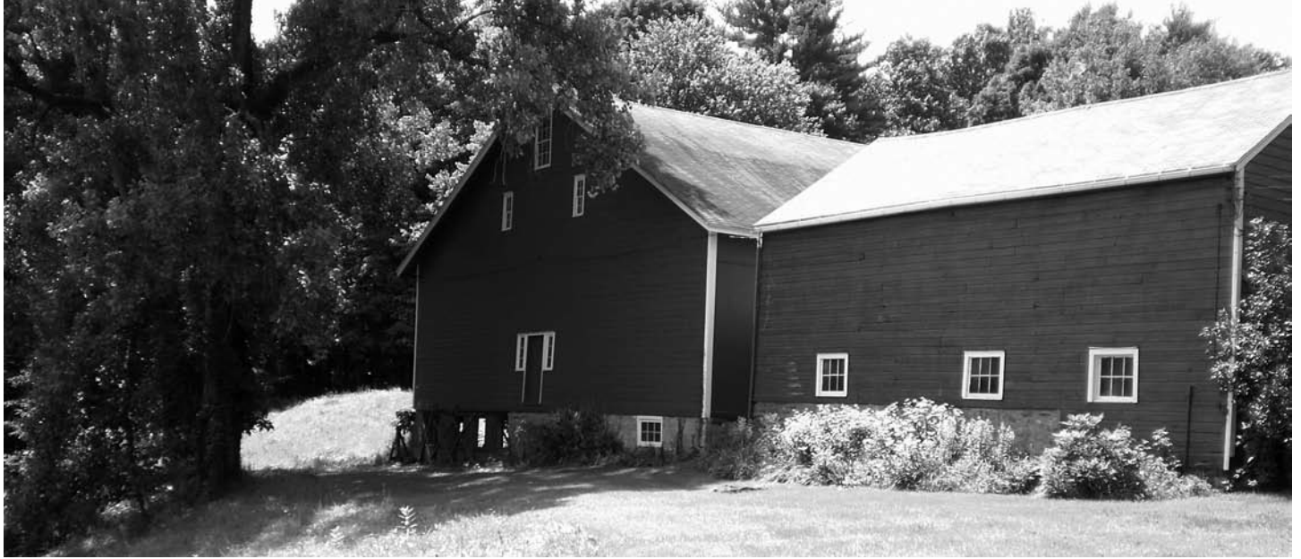
Rear walls of the three-aisle barn at the left and the one-aisle barn at the right are seen in context with the positioning of both structures to the lay
