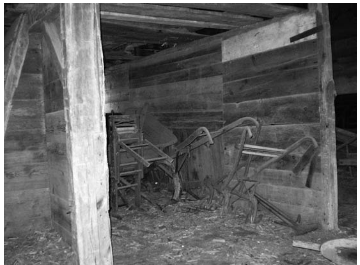
The far end bay in the middle aisle has the unique centered alley that stretches the full width of bay to the far end wall. The alley is framed by posts at each side and south wall of alley consisting of original horizontal boards is seen. Old farm implements are seen in the alley.
