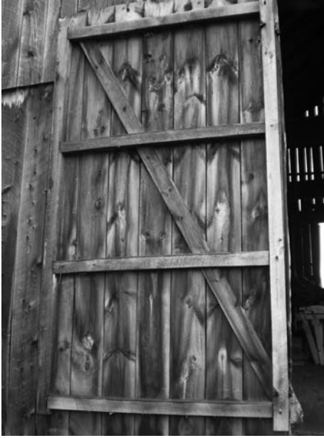
William Bull dendro-dated 1726 three-aisle barn near Goshen in Orange County, New York. View of far end wall with one frame wagon door section is shown.
