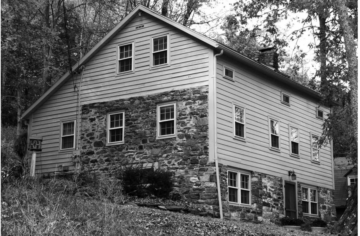
P. Overpaugh House at 172 Clove Valley Road, Town of Rochester
