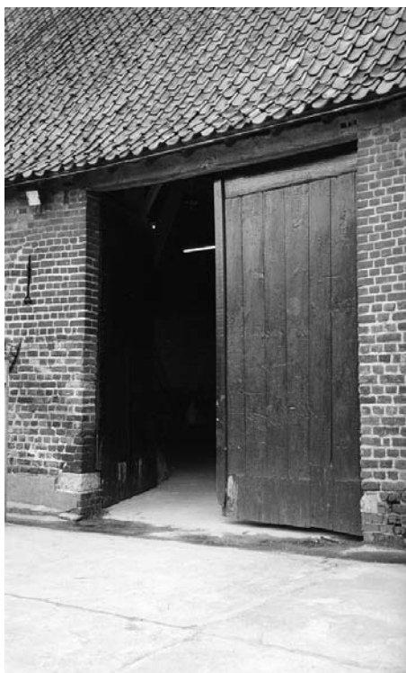
Van Den Bekken farm is located in Kessel area of Limburg near Maas River in the Netherlands. Barn has original frame constructed wagon doors that open into barn. Farm buildings are in court yard arrangement. A date of 1818 in irons is seen on homestead house.
