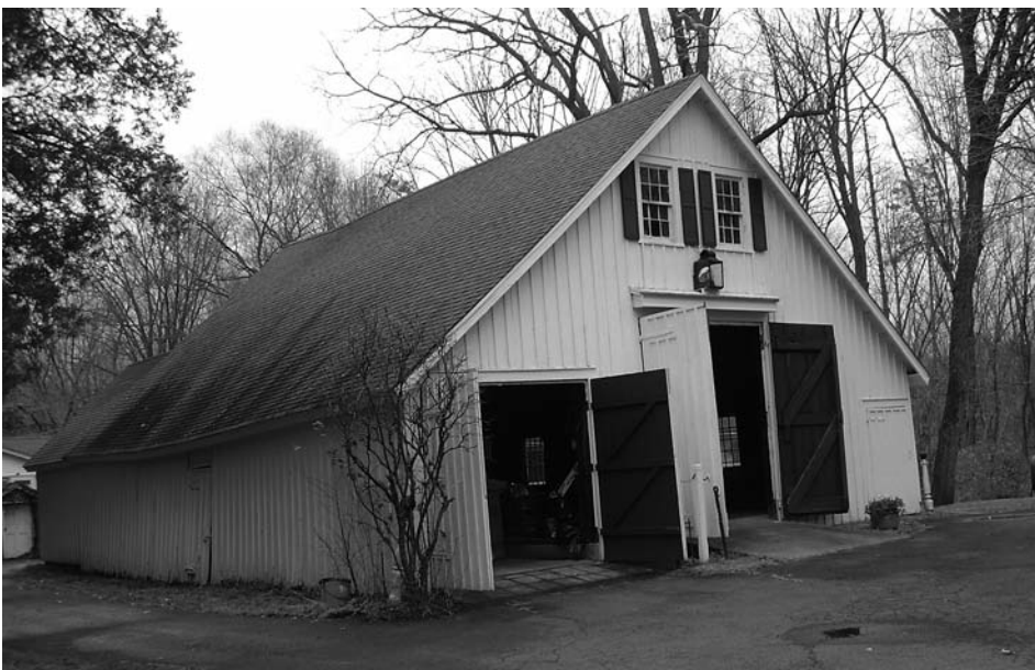
Bartholf circa 1800 three-bay three-aisle barn with one-bay addition is seen on Route 202 in Mahwah, Bergen County, New Jersey. Barn only had one end wall wagon door opening.
