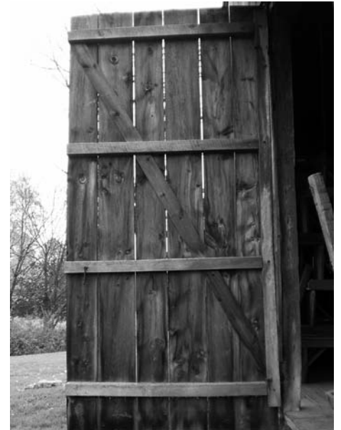
Near end wall of Bull barn is seen with its interior surface of full single height door section. Note four horizontal bars that join to side vertical stile in frame constructed door patterned after possible original wagon doors.
