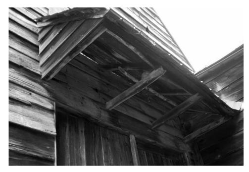
Above: Pentice at end wall of Bogart barn in Marbletown, Ulster County with original arms and non-original rafters. Pentice stretches across full width of wagon doors. Below: Close-up of possible original mittelmanse at end wall wagon doors at Bogart barn. Note how top end of post enters into soffit of end wall anchor-beam. The post in this barn is seen to the exterior of the door while in other barns they are seen inside the wagon doors.
