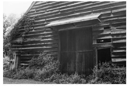
Wemple four-bay three-aisle barn near Schenectady, New York has the most complete set of end wall wagons doors (with wooden hinges) anywhere in Dutch settled areas.
