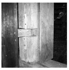
At near end wall of Wemple barn is wagon door post with slot for wooden hinged door. Door that swings on wood pintle is open and has swung into the barn.
