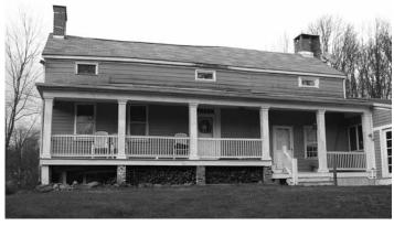
Muller house in Montgomery, Orange County. There is a vertical seam between the right & center eyebrow window. To the right of the seam is claimed to be built in 1724.
