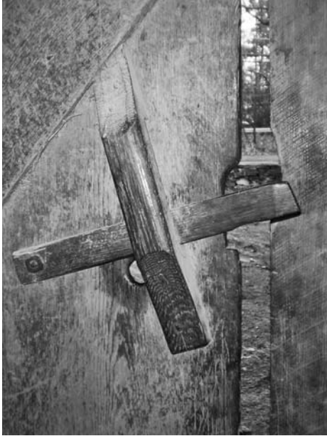
Close up of two-piece all wood door-latch in interior placed wagon doors seen in John Snyder side wall entry barn. Note quite severe angle of door-latch keep.
