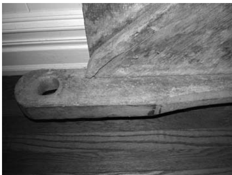
View of one end wall wagon door of Oliver barn that shows flared condition of wooden hinge.
