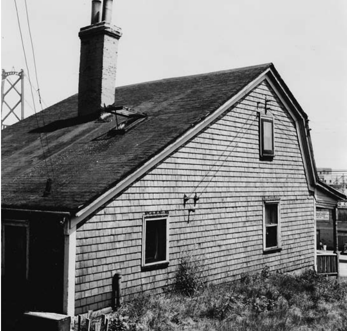
Side view of the Burge House.
