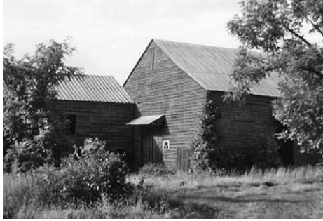
DuBois probable three-bay three-aisle barn that was formerly located on Libertyville Road near New Paltz in Ulster County. This barn had both an end wall wagon door with wooden hinges and perhaps uniquely a side wall wagon entrance with wooden hinges.
