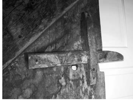
View of two piece door latch of one end wall wagon door section formerly part of Oliver barn. Both wood pieces are oak. Circular finger hole is barely visible below latch.
