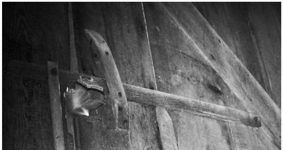
Interior of original end wall wagon doors at the Bogart barn with close-up view of unusual four piece all wood door latch release mechanism. Door was unlatched in interior of barn.
