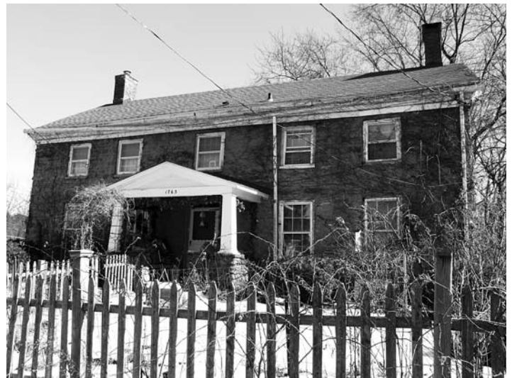
At the corner of Teetsel Street and Ulster Avenue (Rt. 32), is this Georgian style stone house said to be built in 1763. Is this the house of Johannes Myer?
