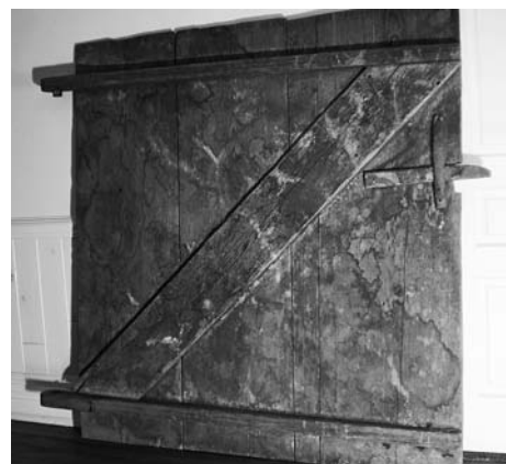
View of one end wall wagon door section – formerly part of Oliver barn on Route 209 in Marletown, Ulster County – showing the door that includes two wooden door hinges, diagonal batten and four front face vertical boards.
