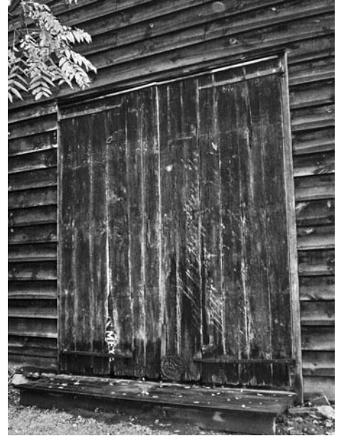
Wagon doors seen at the Hopper-Goetschuis Museum barn in Saddle River, Bergen County, New Jersey. These re-cycled doors were found at a former site in a side entry Dutch-Anglo barn that stood on another road in town.
