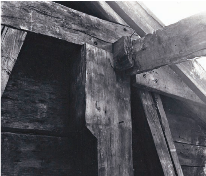
Detail of the Burge House framing joint, circa 1968.
