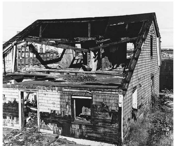
The Burge House after a fire in 1968.
