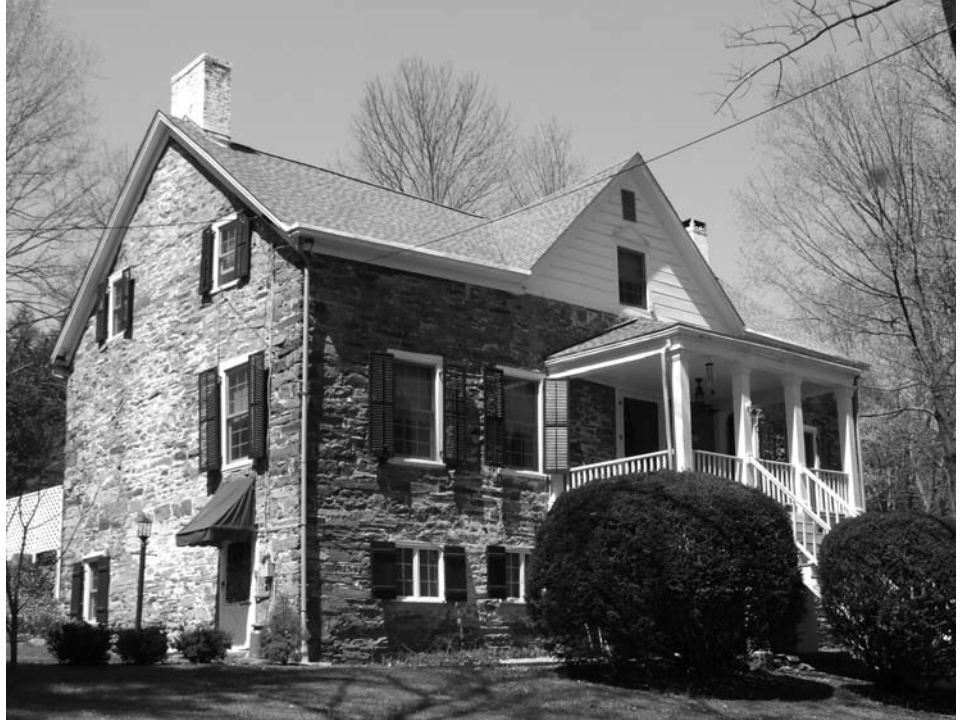
Seen on Sawkill Ruby Road, this unidentified house is a typical Ulster Co. stone house except for the ground level cellar.
