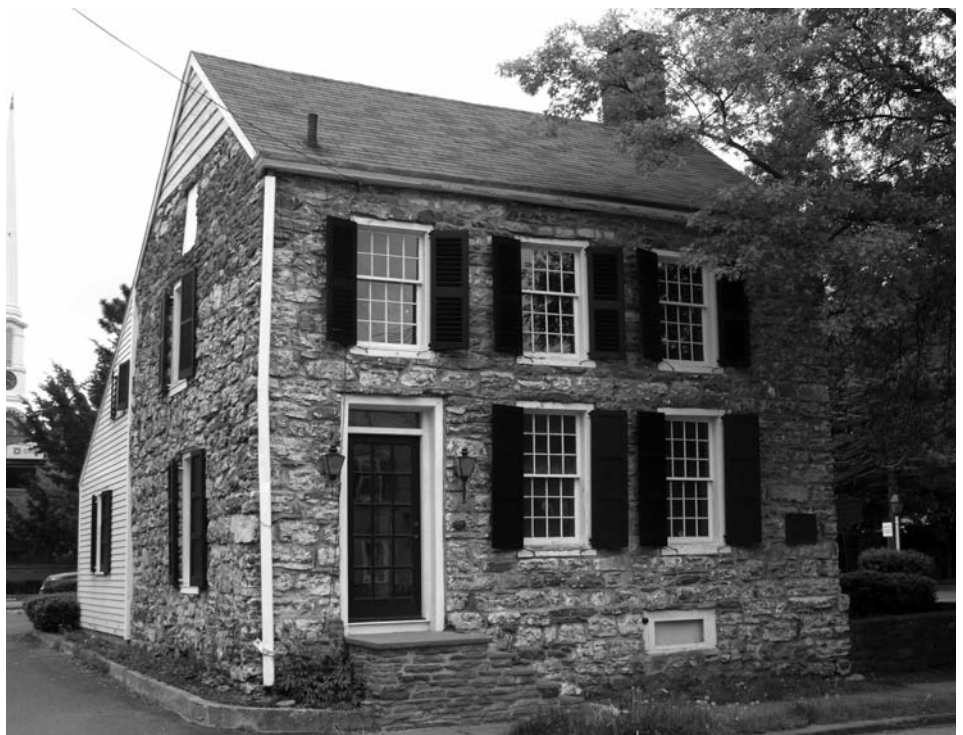
For many years known as the Cornelius or Christopher Tappan house, the cellar is of the Gysbert Vanderburgh house on which Abraham Hasbrouck, Jr. erected the current structure after the British burned the original house in 1777.
