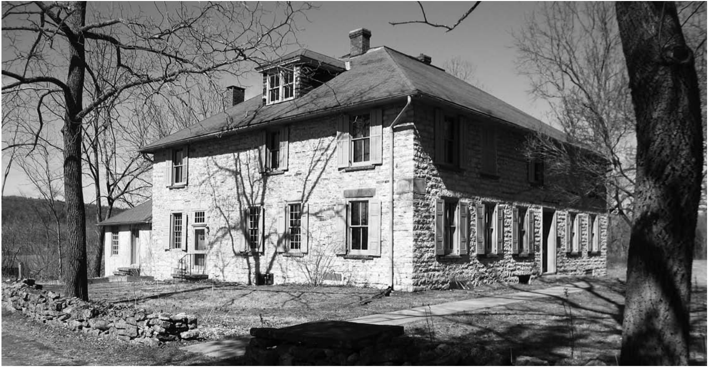
Figure 1. Bevier House, Marbletown, New York. Current conditions reflecting additions and alterations made in the nineteenth century. The house is owned by the Ulster County Historical Society (Photograph by Neil Larson, 2005).
