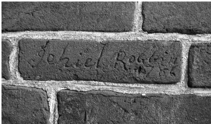
Fig. 4 Photograph of remaining fragments of original vining and penciling at the Payne house in Fort Miller, Washington County, New York. Jehiel Robbins was the brick mason for the house, constructed in 1786-1787.
