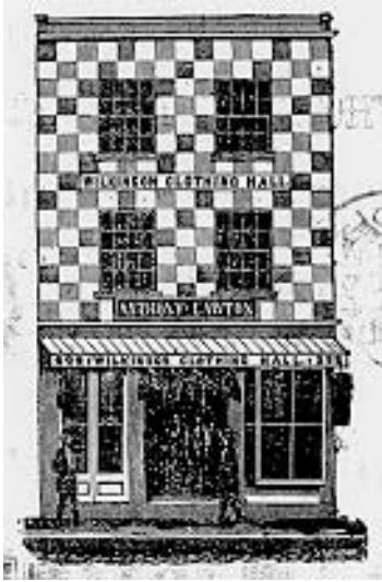
Fig. 2 "Wilkinson Clothing Hall," a commercial building on River Street in Troy, NY, painted in the 'harlequin' or 'particolored' style in 1850.
