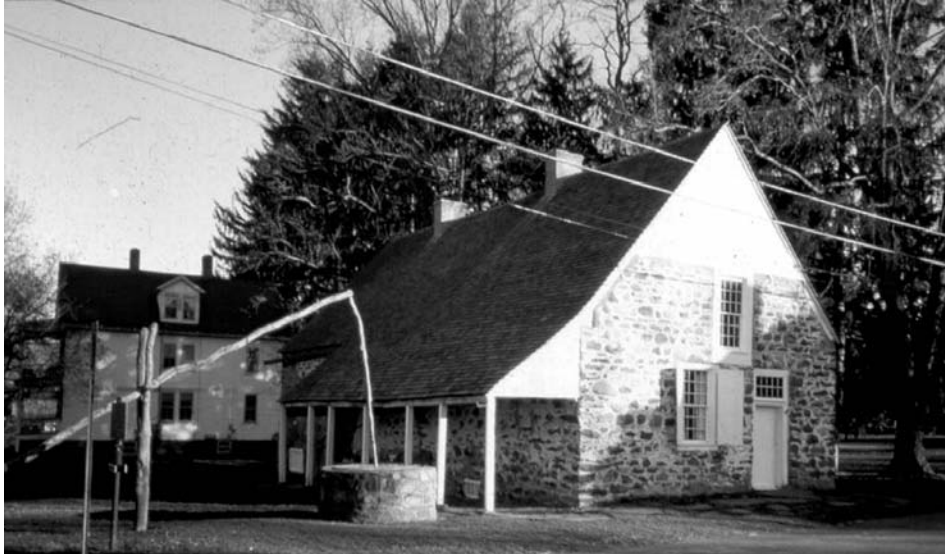
Figure 4. Bevier-Elting House, New Paltz, New York. One of a very few houses surviving in New York with its front gable façade intact. (Photograph by Neil Larson, 2004)
