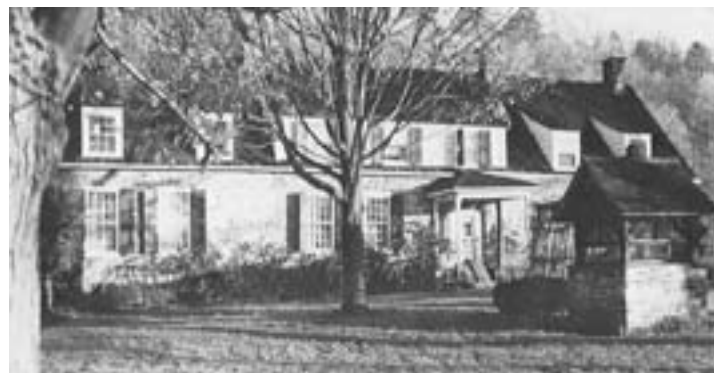
Fig. 5 – Andries DeWitt house, mid-18th-century, Hurley Mountain Rd., Lamontville. Photo from Early Architecture in Ulster County, 1974 . First floor plan, measured and sketched by T. Ryan.
