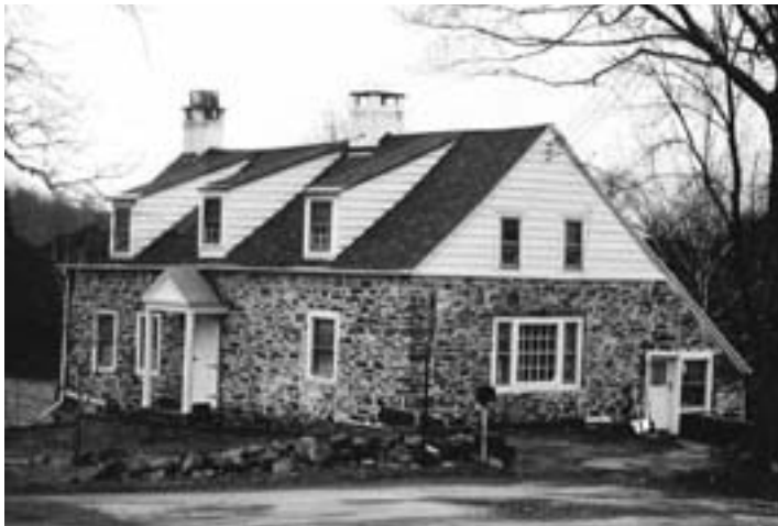
Fig. 4 – Gerrit Van Wagenen house and outlet, mid-18th century, Berme Rd., Marbletown. Photo by T. Ryan.
