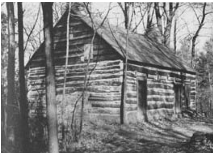
Fig. 3 – Adam Yeaple house, ca. 1770, Mohonk Mountain Rd., Aligerville. Photo from Early Architecture in Ulster County , 1974.
