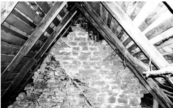
Fig. 8 – Detail of interior wall in Cornelius Cool House, Hurley, NY, showing evidence of brick vlechtingen in stone gable. Photo by Jim Decker, 2012.
