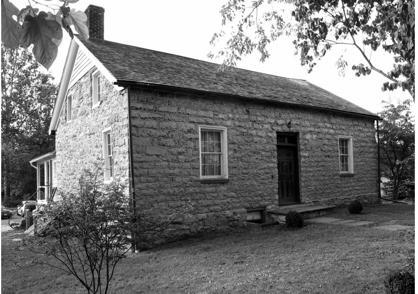
Fig. 1 – View of Henry Brodhead House from southeast. Photo by Neil Larson.
