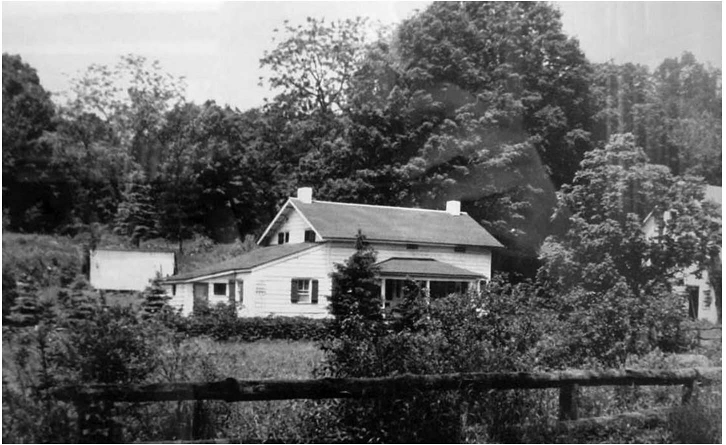
Fig. 2 – Historic view of house from southeast, c. 1920. The section to the left of the entrance represents an addition, at which time an entire new roof was added. The shed roof extension, containing a kitchen, was added later still.
