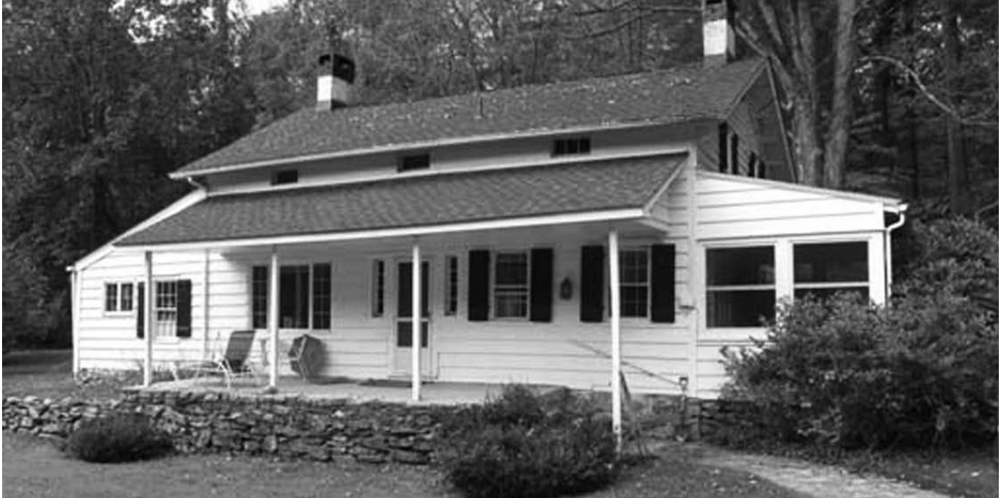
Fig. 1 – Current view of house from northeast. The north section of the front façade containing the entrance and two small windows to its right represents the extent of the original dwelling.
