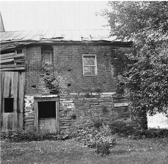
Fig. 2 – East elevation of the North House. September 1969.
