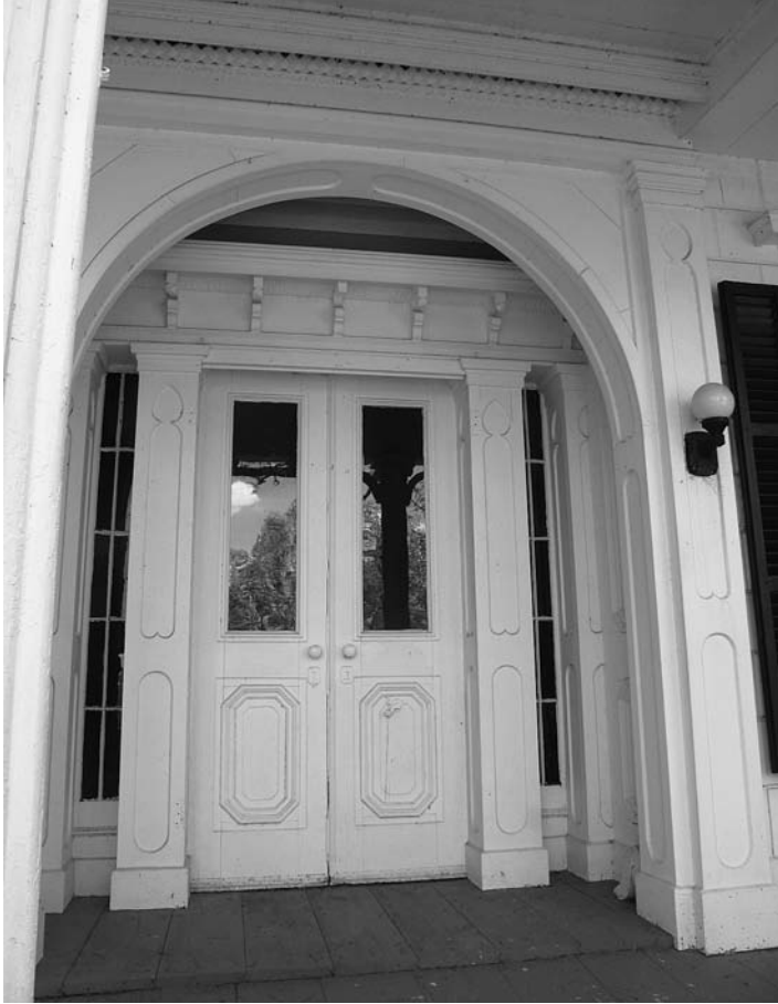
Fig. 8 – Shultz House, entrance detail
