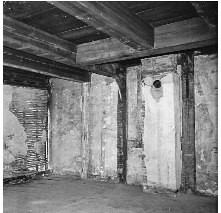
Fig. 8 – Interior of the first floor of the North House looking towards its north-west corner. Note the whitewashed wall post that has a channel cut down the middle of it to hold the bricks of an original partition. Note also the stove chimney in front of an original window frame and the header installed in the second floor framing to make an opening for the smoke hood of a basement fireplace on the north wall. At the right side of the photo can be seen the slanted line of the east side of the former smoke hood which was replaced in 1878 by the stove chimney. October 1969.
