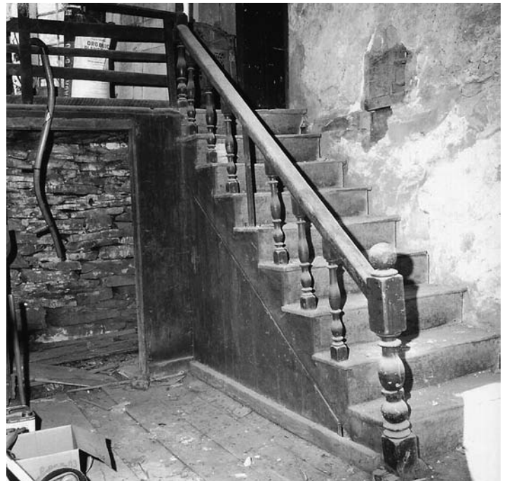
Fig. 4 – Interior of 'connector' with a re-used stair from an unknown source set up against the south wall of the North House. Note the exploratory opening made in the wall to reveal constructional details. October 1969.
