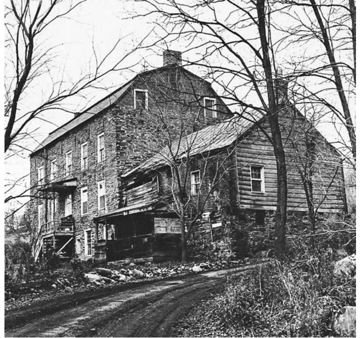
Fig. A – View of Coeymans mansion and North House from the north east. November 1967. Photos by J.R. Stevens.
