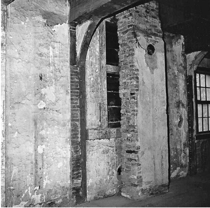
Fig. 9 – Like the last photograph, this shows the stove chimney in front of the 'kloosterkozijn' frame. Within the window openings can be seen the inside of the weather boarding installed at the end of the 18th century. October 1969.
