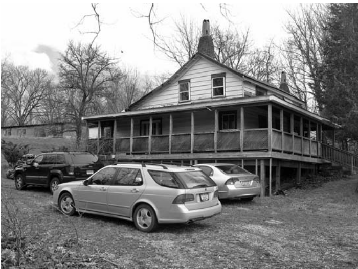
Kimlin House from SE.
