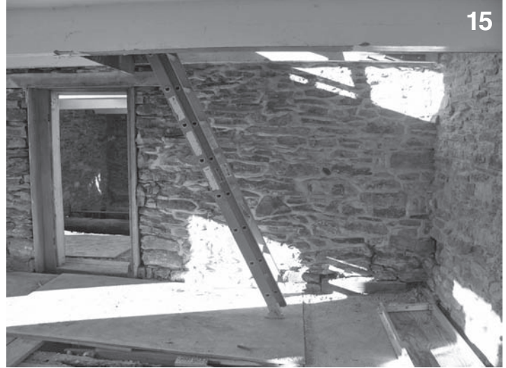
Fig. 15 – Interior view of stone wall dividing two sections of the house, 2013. The doorway is centered in the wall and retains its original 18th-century dimension and materials. However, the wall is overly thick, with ledgers recessed into both sides and not precisely aligned with seams in side walls and roof plates. It appears that this wall was reworked when the second section was constructed including the placement of the doorway. The stair location in the northeast corner of the south room seems to be historically appropriate, but ceiling boards have been removed in the north end and with it any potential evidence of a stair or ladder space in the original house.
