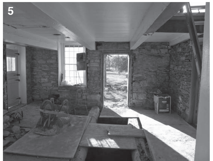
Fig. 5 – View of interior of south section looking west, 2013. Exposed stone walls and door and window framing appear to be intact. A heavy lintel spans the door opening and the window is neatly placed between ceiling beams. Note floor beams, which are logs flattened on the top for flooring, and finished beams and boards in the ceiling. The doorway on the left side of the image is in the gable end facing the street. The hole for the stairs is partially visible in the upper right corner of the view; the stairs and their enclosure were removed.
