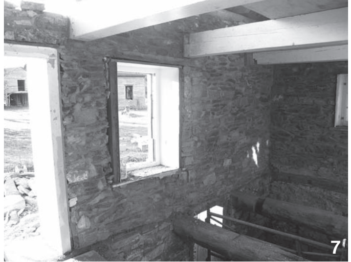
Fig. 6 – Detail of west wall, 2013. Door and window openings in what appears to be the original house built c.1722. The window opening was reduced in size probably when a casement window was replaced with a sash unit. The door appears to have been a still later addition, possibly cut through when the balloon-frame wing was added. The interior stone wall between the two sections is nearly flush with the right side of the doorway, which would align its exterior face with the seam.
