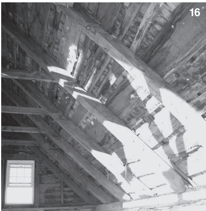
Fig. 17 – View of rafters in south section of house, 2013. No distinction can be made between the roof systems in the two sections suggesting that the entire roof was built in 1752.
