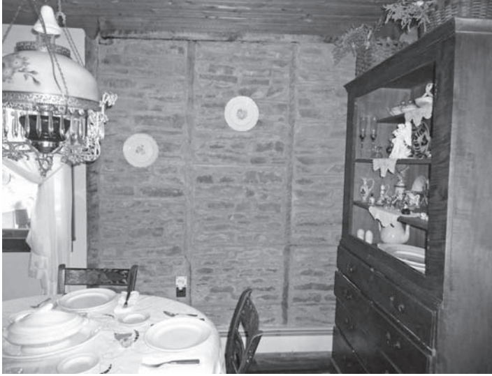
Fig. 4 – Van Wagenen-Krom House. Interior view showing original timber frame and stone nogging.
