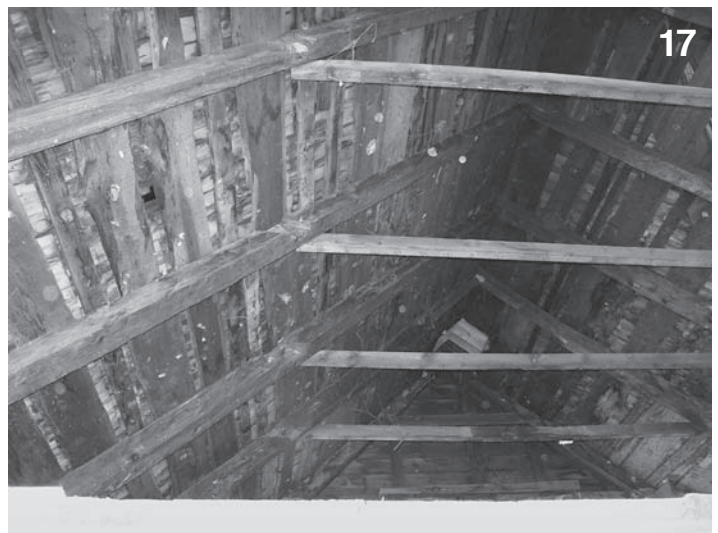
Fig. 17 – View of rafters in south section of house, 2013. No distinction can be made between the roof systems in the two sections suggesting that the entire roof was built in 1752.
