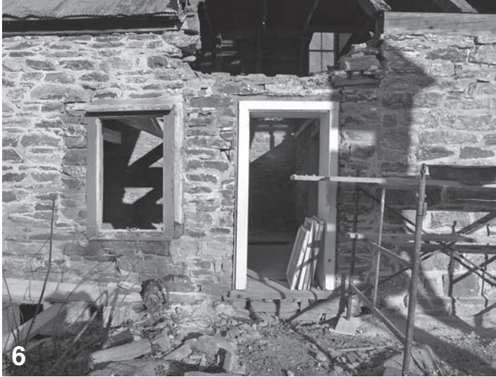
Fig. 6 – Detail of west wall, 2013. Door and window openings in what appears to be the original house built c.1722. The window opening was reduced in size probably when a casement window was replaced with a sash unit. The door appears to have been a still later addition, possibly cut through when the balloon-frame wing was added. The interior stone wall between the two sections is nearly flush with the right side of the doorway, which would align its exterior face with the seam.
