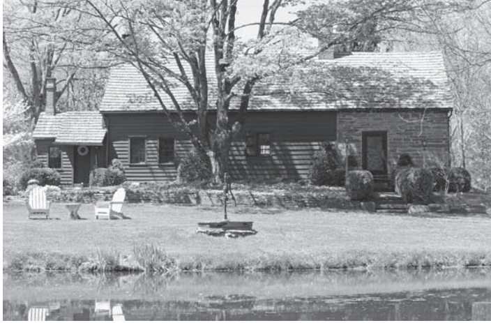
Fig. 6 – Hendrick Smit House. One of the oldest H-bent timber-framed residence in the Hudson Valley. Its construction remains a mystery after an extensive and poorly documented “restoration.”
