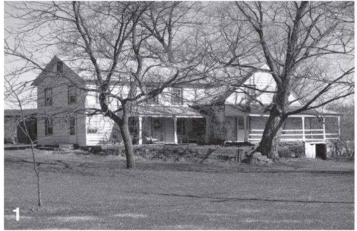
Fig. 1 – View of Osterhoudt house from southwest, 2010.
