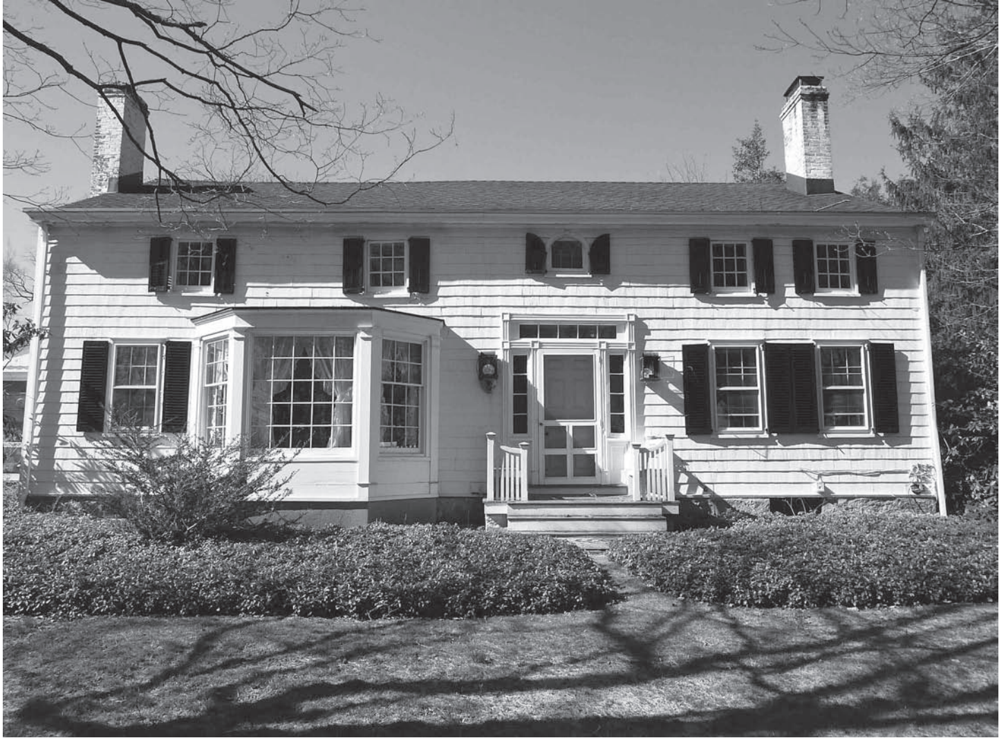
Fig. 3 – House at Hallock's Mill, view of south façade. The three-bays and entrance on right side represent the dimensions of the original house. Photo by J-F Delaperouse.
