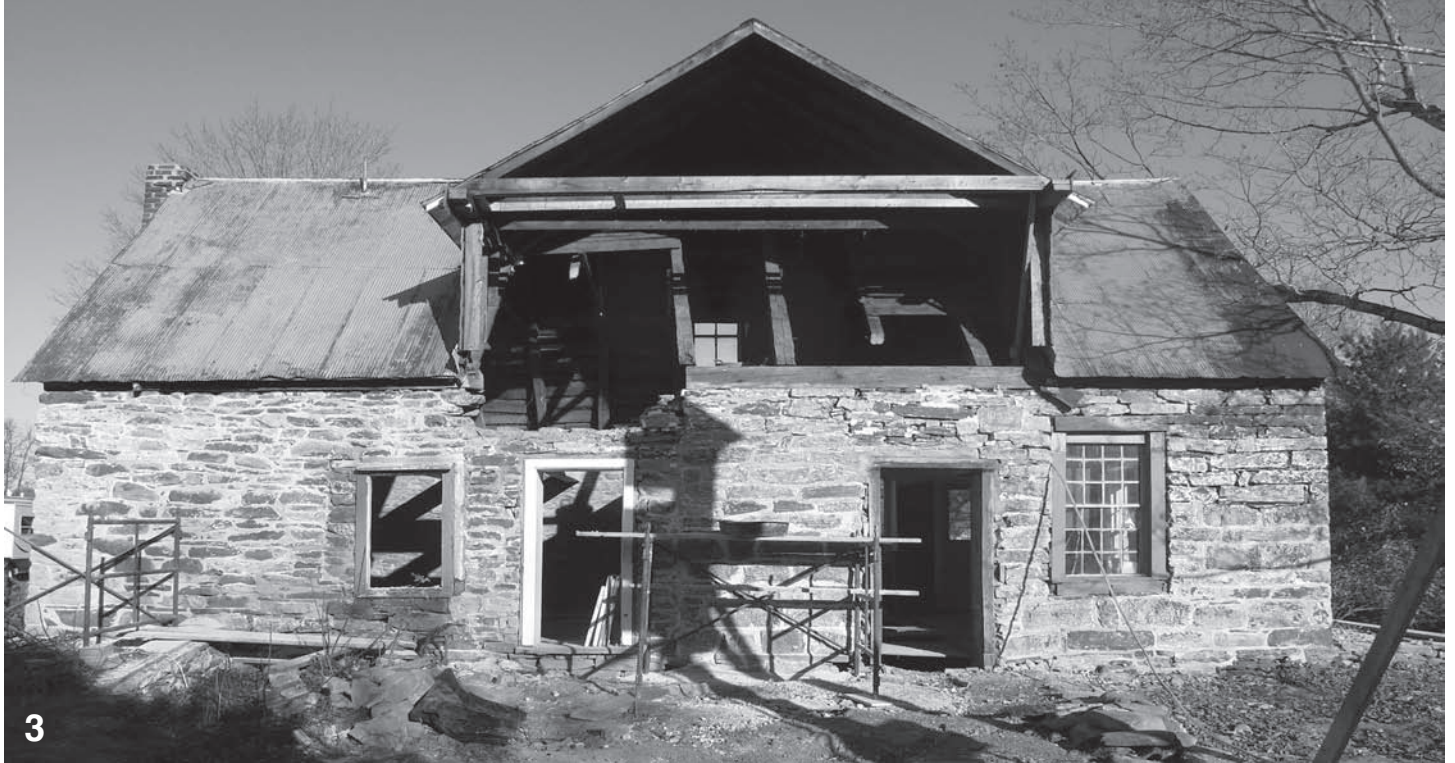
Fig. 3 – View of house from west, 2013. Seam between two sections visible in shadows to right of left door. Note larger stones and more even coursing on right side where door and window openings appear intact unlike openings on left side, which have been altered. View also shows roof framing of demolished addition.
