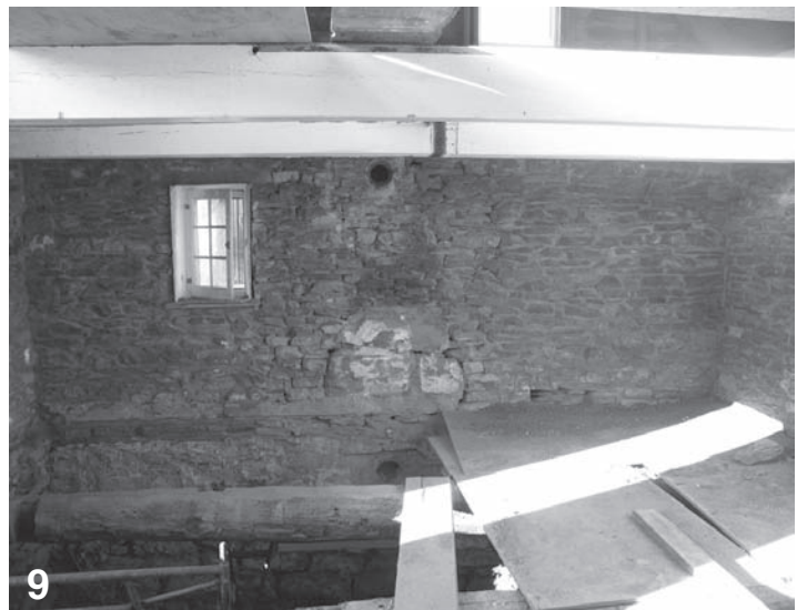
Fig. 9 – Interior view of north room from south, 2013. The casement window opening with its wood lintel appears to be intact. Evidence of a firebox back from a hearth later removed is visible at floor level in center. Trimmers surviving in ceiling and pockets in floor beams, as well as a shelf in the basement wall that once supported cribbing, all point to the prior existence of a jambless fireplace.
