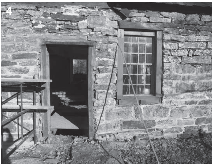
Fig. 5 – View of interior of south section looking west, 2013. Exposed stone walls and door and window framing appear to be intact. A heavy lintel spans the door opening and the window is neatly placed between ceiling beams. Note floor beams, which are logs flattened on the top for flooring, and finished beams and boards in the ceiling. The doorway on the left side of the image is in the gable end facing the street. The hole for the stairs is partially visible in the upper right corner of the view; the stairs and their enclosure were removed.
