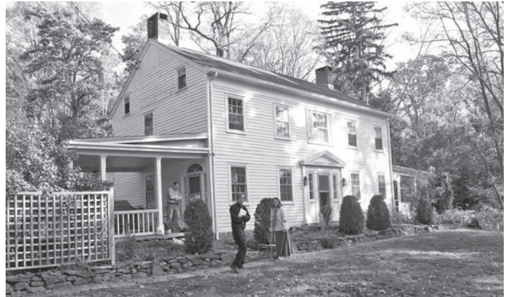
Fig. 1 – View of Tompkins-Scribner House from southwest. Photo by N. Larson.
