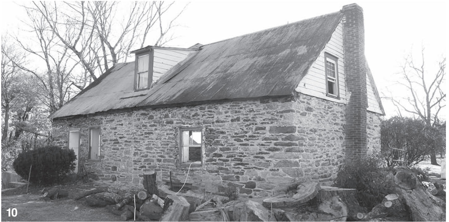
Fig. 10 – View of house from northeast, 2013. The east wall of the house contains an added window in the north section and an added doorway in the south section. From the stonework, it does not appear that the c.1722 house had any openings on the east side. The window opening near the doorway appears to be in its original dimensions. Like the window on the opposing side of the room, it is positioned between beams on the interior. Unlike the windows in the original house, the windows in the 1752 addition were sash units. The seam between the two sections is visible in the center and the lintel for the original basement entry is just discernible under the window on the right and behind the tree parts. It was filled in with stone when a new door was created on the west side of the house.
