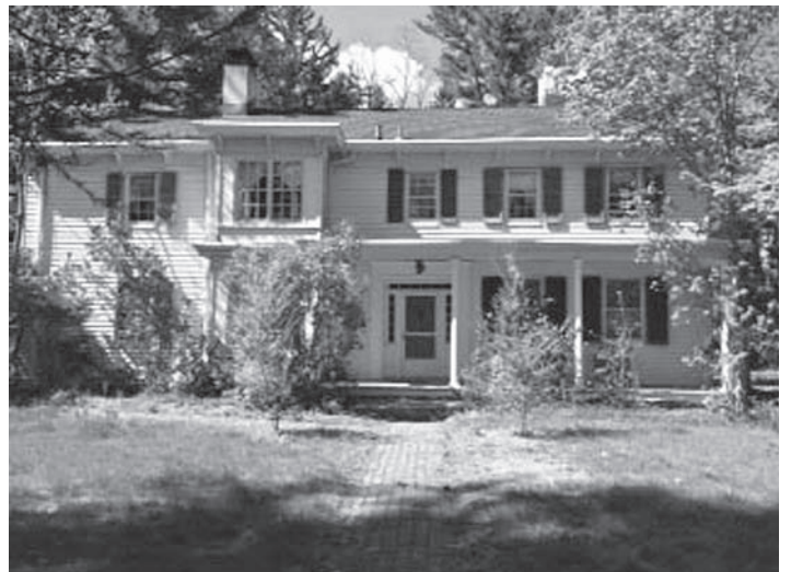
Fig. 4 – Henry Strang House, view of south façade. The three-bays and entrance on right side represent the dimensions of the original house. Photo by J-F Delaperouse.
