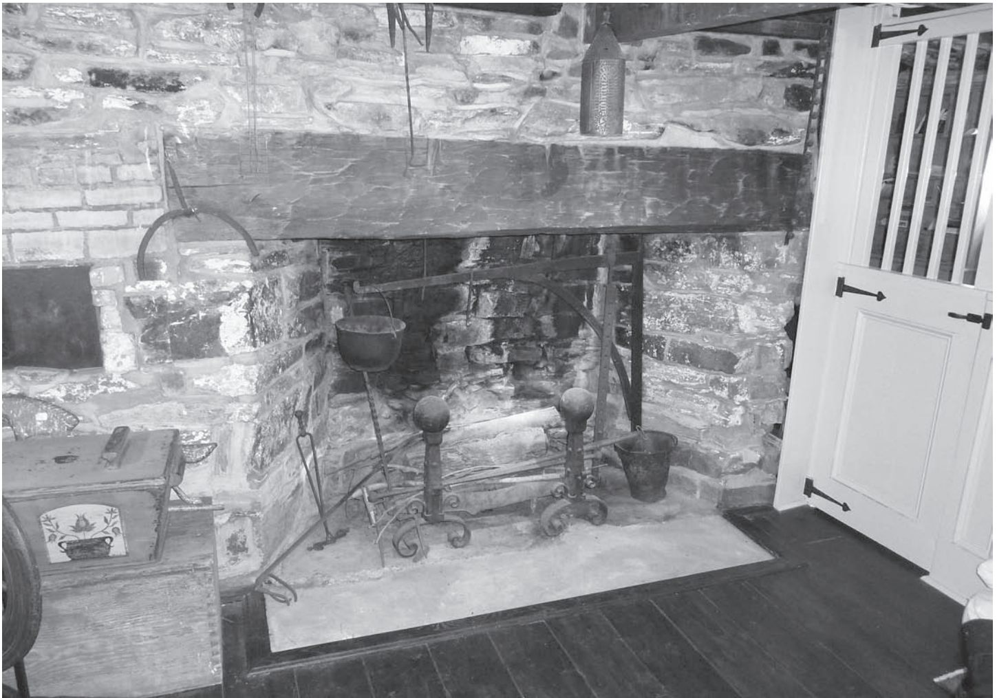
Fig. 2 – House on Croton Heights Road, basement fireplace. Photo by J-F DeLaperouse.
