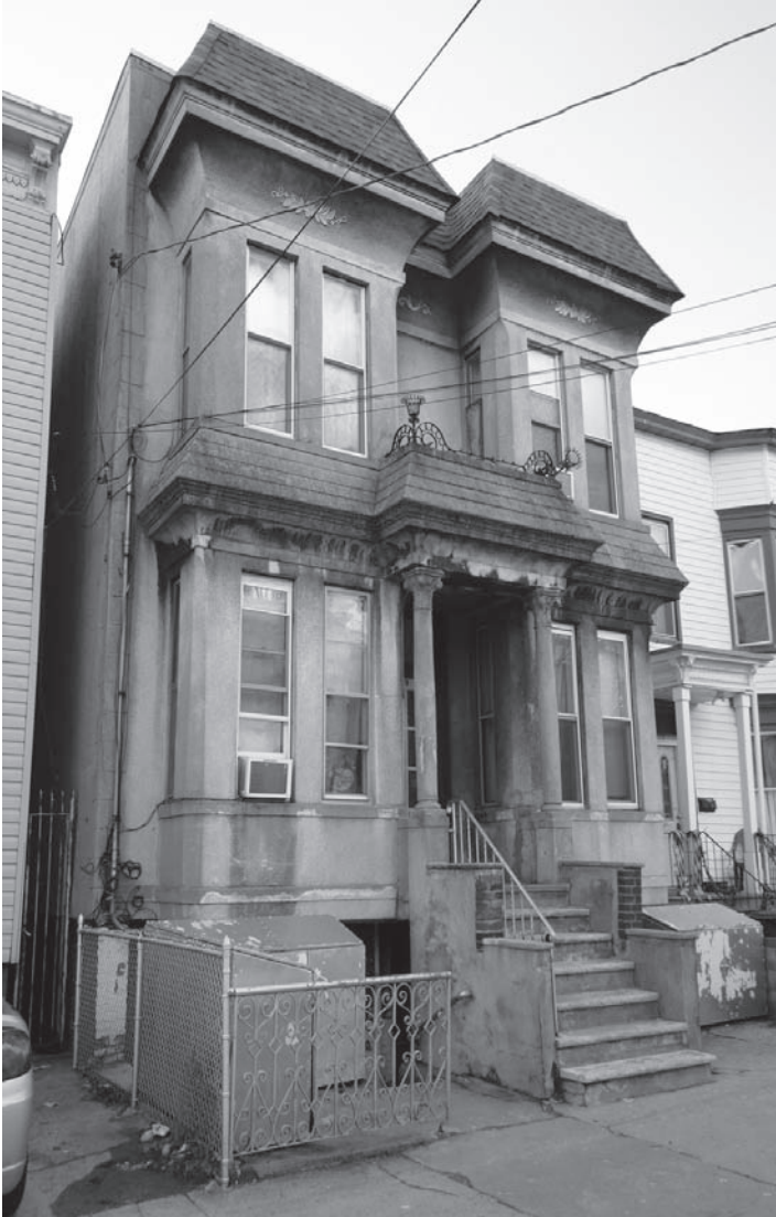
Concrete house on Lincoln St., Jersey City, Bergen County, New Jersey – April tour
