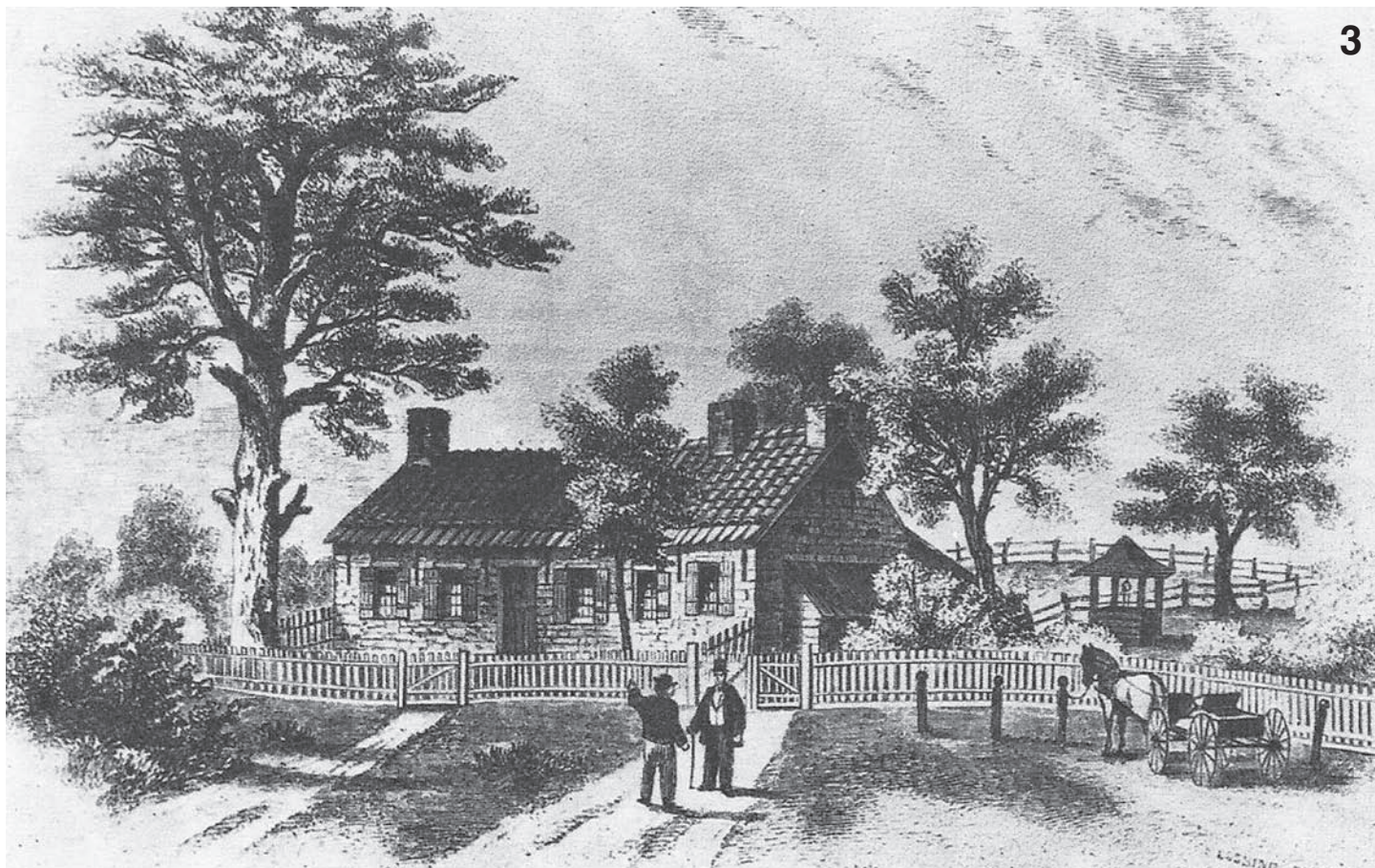
Pl. 3 – Nicasius de Sille, New Utrecht, Long Island 1657, demolished in 1850.
