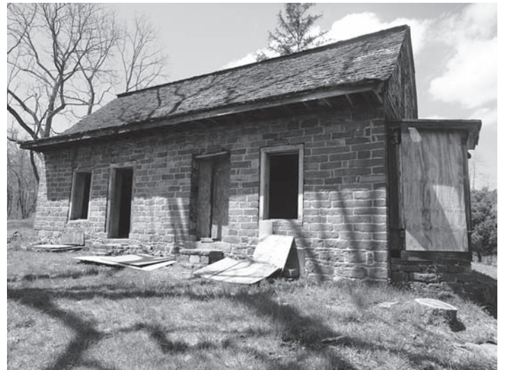
Vanderbilt-Budke house, Bardonia, Bergen County, New Jersey – April tour
