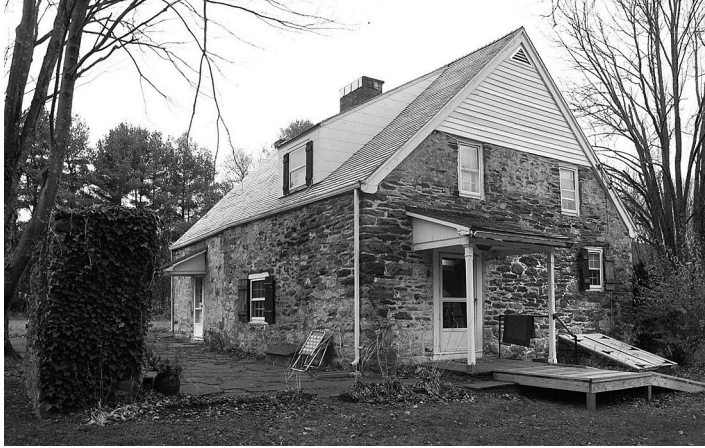
Fig. 1 – View of house from southwest. Photo by Neil Larson.
