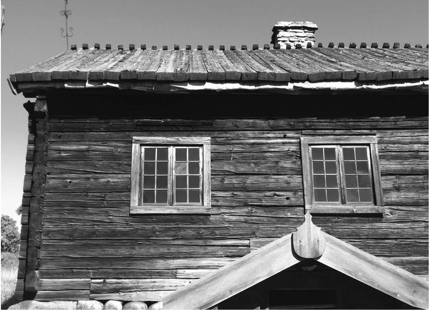
Fig. 4 – Detail of log wall and plank roof construction, Skansa Museum. Photo by Neil Larson, 2015.
