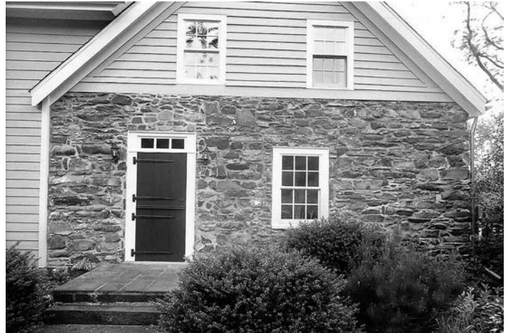
Fig. 9 – View of Du Puy House from east. Photo by author.
