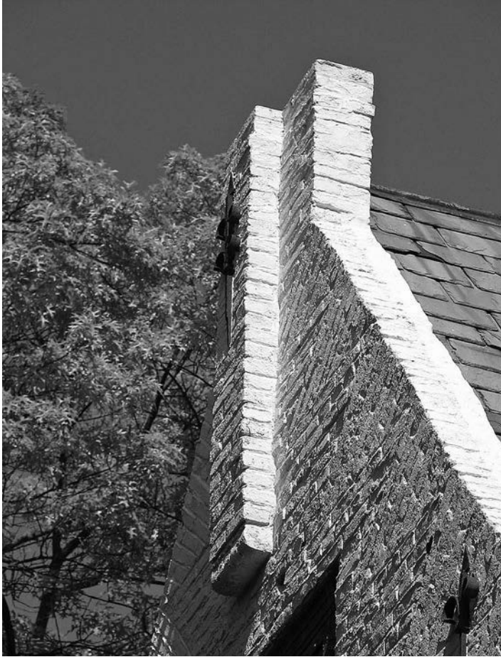
Fig. 7 – Detail of the spout gable on the Yates house in Schenectady (Author's photo, 2008).
