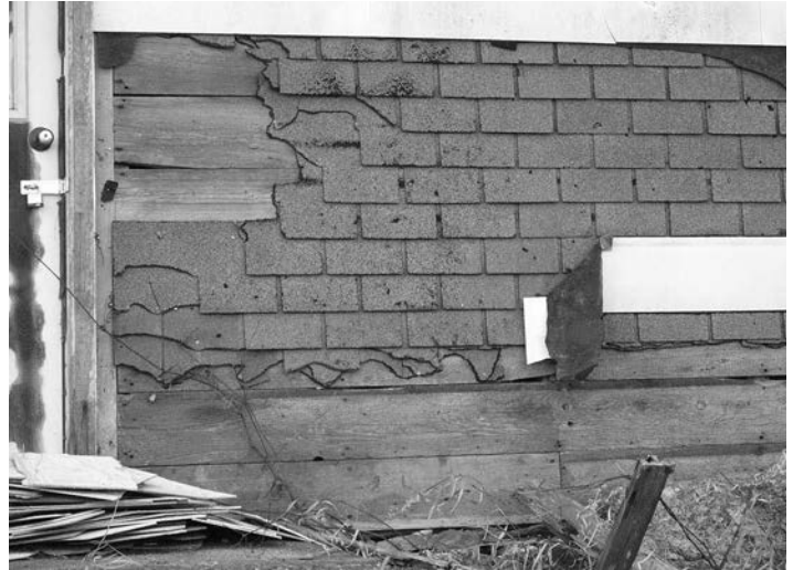
Fig. 13 – Detail of siding layers on north end of kitchen ell. Photo by Neil Larson, 2015.
