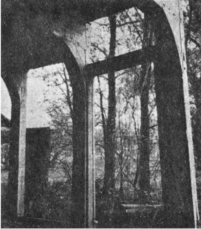
Fig. 6 – View from of the north range of anchor beam posts, corbels and anchor beams, ca. 1914. From Percy M. Van Epps, Contributions to the History of Glenville (1926).
