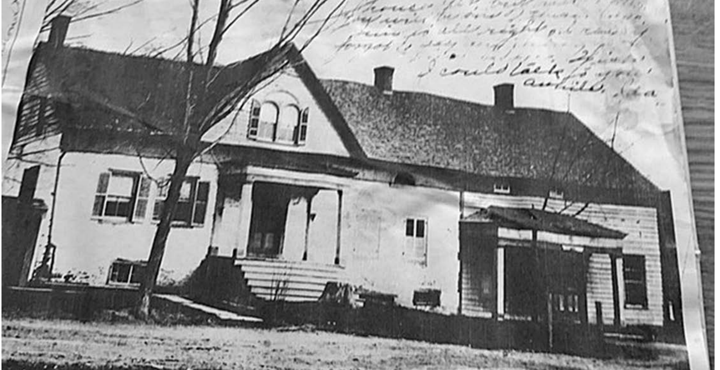
Fig. 5 – View of house from south. Photo ca. 1900. Courtesy of Juliette Bennett. The wood frame extension was added for the store in the 1870s.
