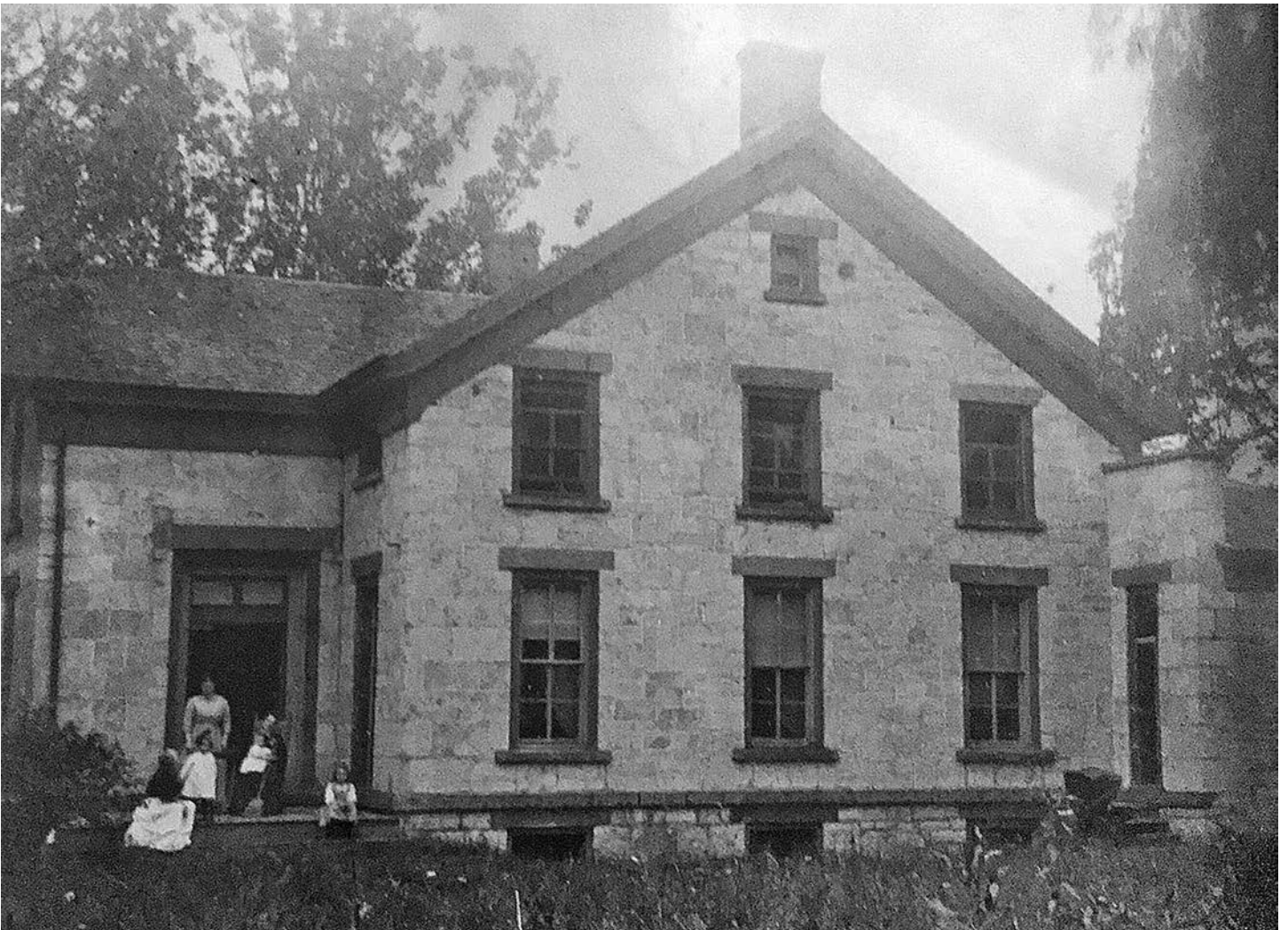
Fig. 4 – Historic view of house from south, ca. 1900. Photo courtesy of Joy Pollock.
