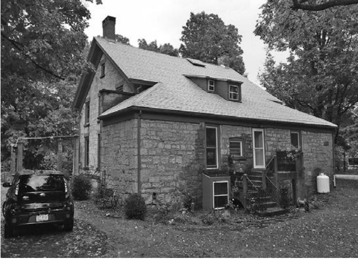
Fig. 3 – View of house from southeast. Photo by Neil Larson.
