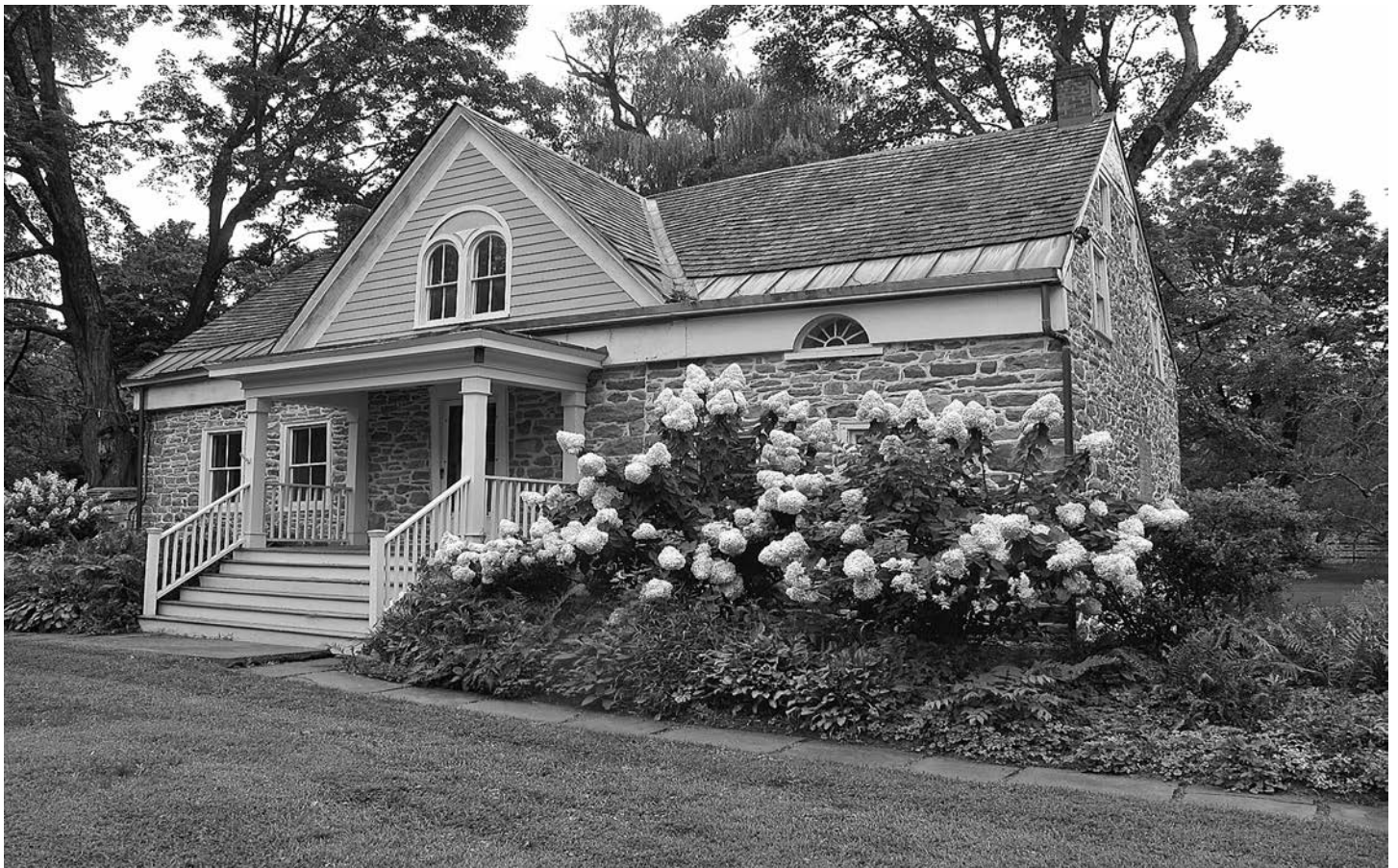
Fig. 1 – View of house from south. Vertical seam visible to left of tallest flowers. Photo by Neil Larson, 2018.
