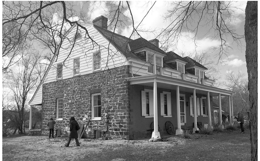
Fig. 1 – View of Schuyler-Colfax House from SE. Photo by Neil Larson, 2019.
