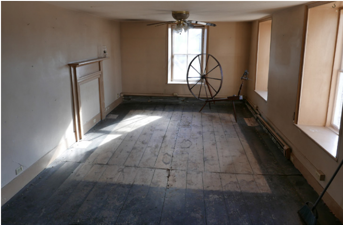
Fig.6: Front (best) room on first-floor from the passage. The mantel was the backdrop for a freestanding coal stove. The partition between the stair hall and best room has been removed.
