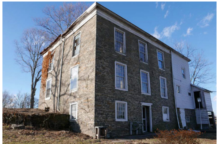
Fig.3: View of house from SE.
