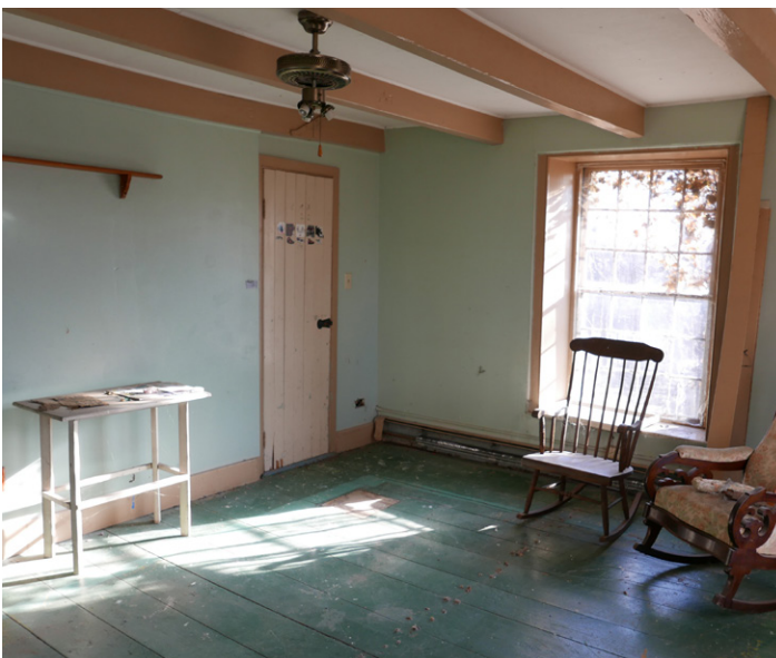
Fig.7: Front bed chamber on second floor with exposed beams on ceiling.
