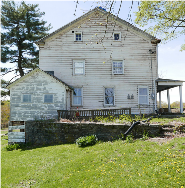
Fig.8: The north elevation of the 1870s frame addition.
