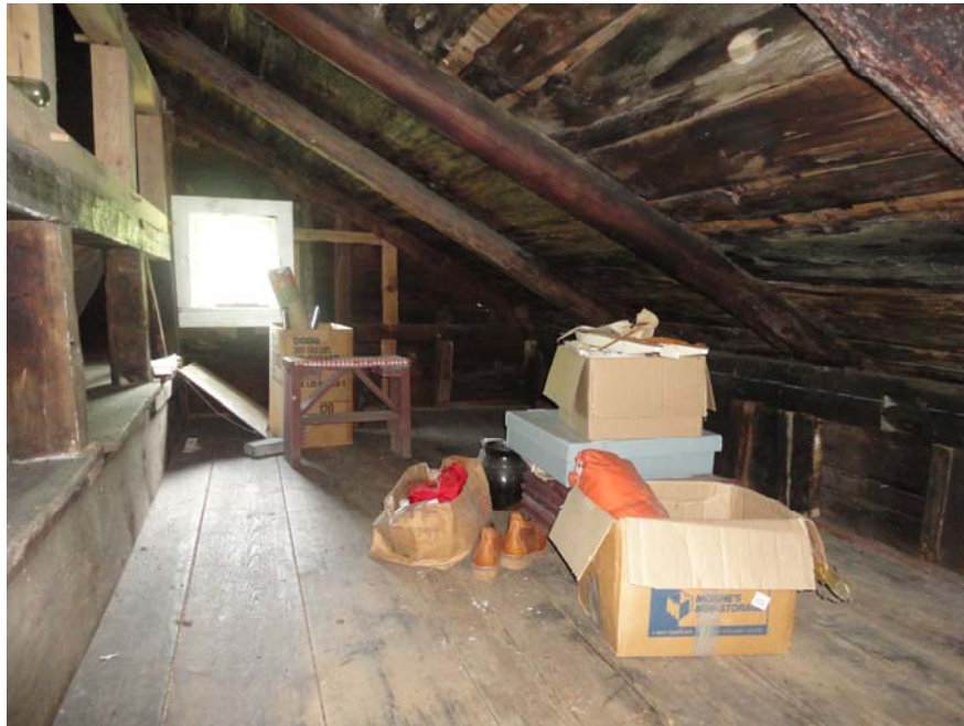
Photo 10. View looking west, in the leanto, second floor, July 2012.
