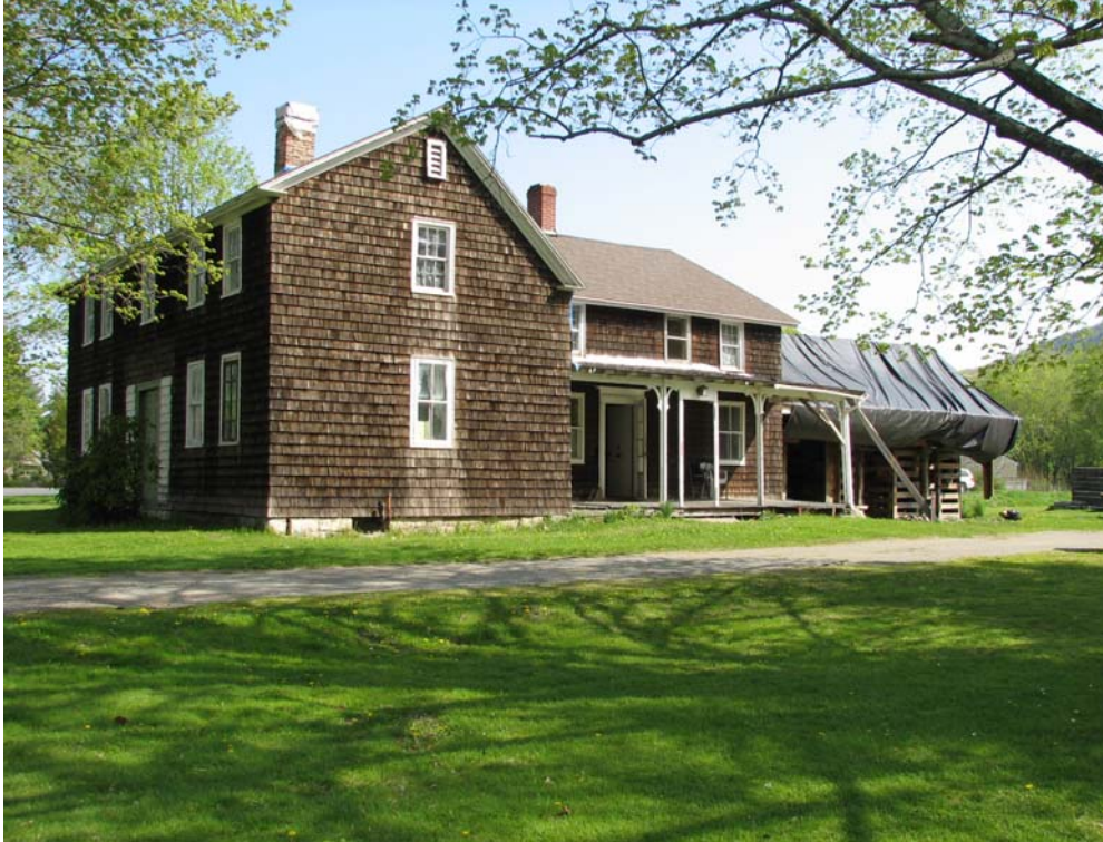
Photo 4. The house as it appeared in May 2010, looking northeast.
