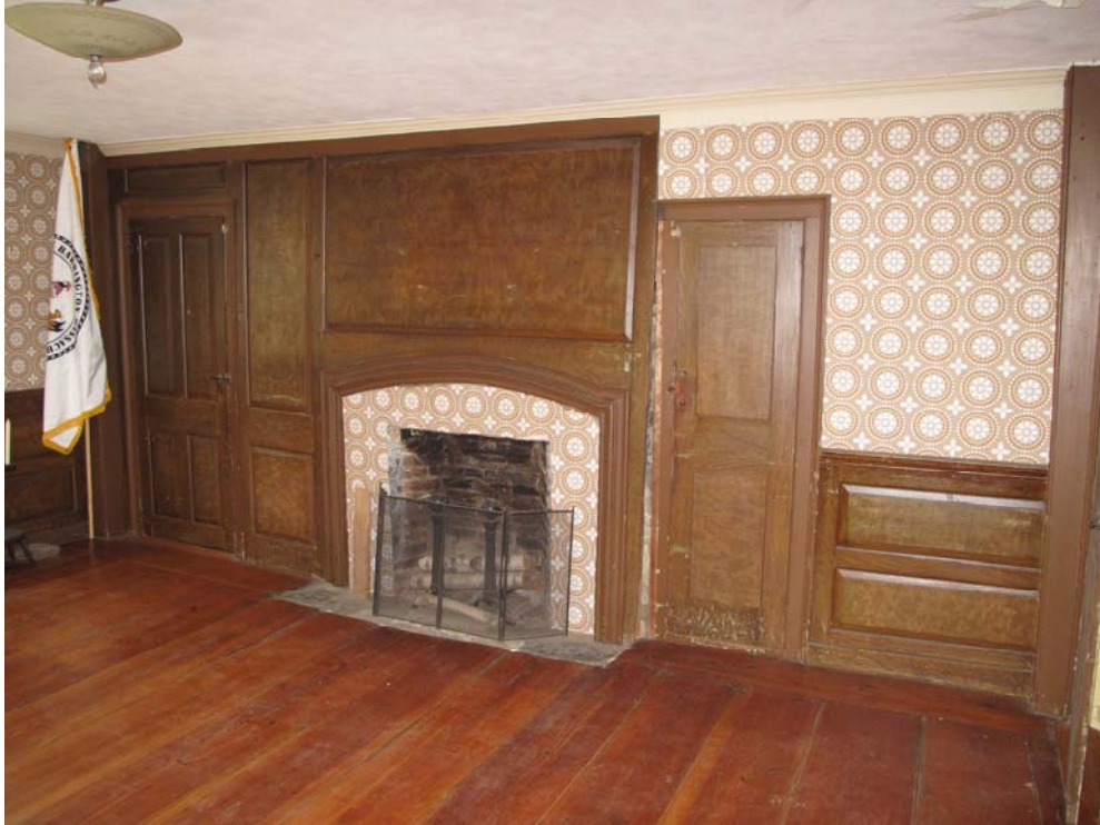
Photo 6. Paneled wall and wainscot in the south parlor, looking north-northeast, 2010.
