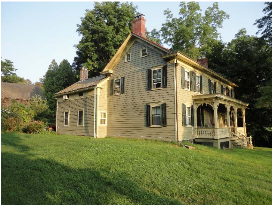
Figure 6. 706 River Road, looking southeast, 2014.
