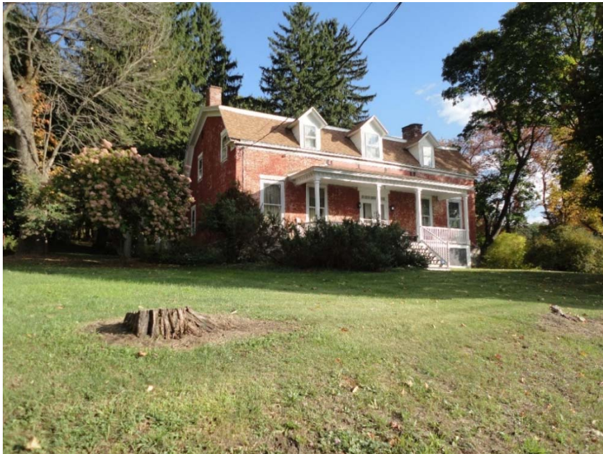
Figure 3. 680 River Road, looking east-southeast, 2014.
