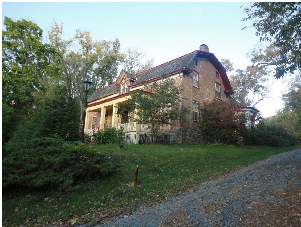
Figure 10. 732 River Road, looking east-northeast, 2014.
