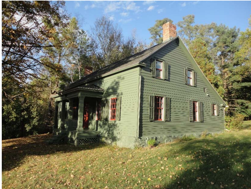
Figure 8. 712 River road, looking northeast, 2014.
