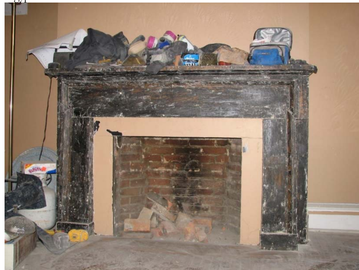
Painted wood mantle in first floor of 2 Franklin Place.
