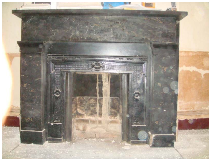
“Egyptian” marble mantle in first floor of 3 Franklin Place.
