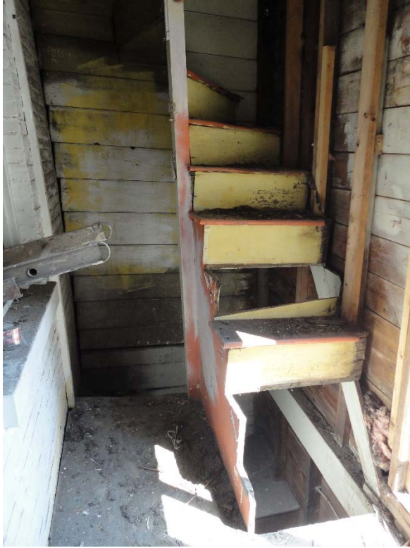
Service stair in 3 Franklin Place, previous to its removal.
