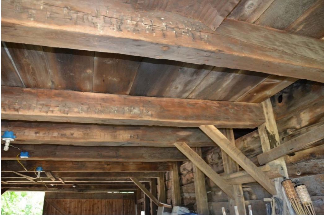
Figure 8. The closely-spaced bents of the Peck barn (photo by W. Wheeler, 2010).
