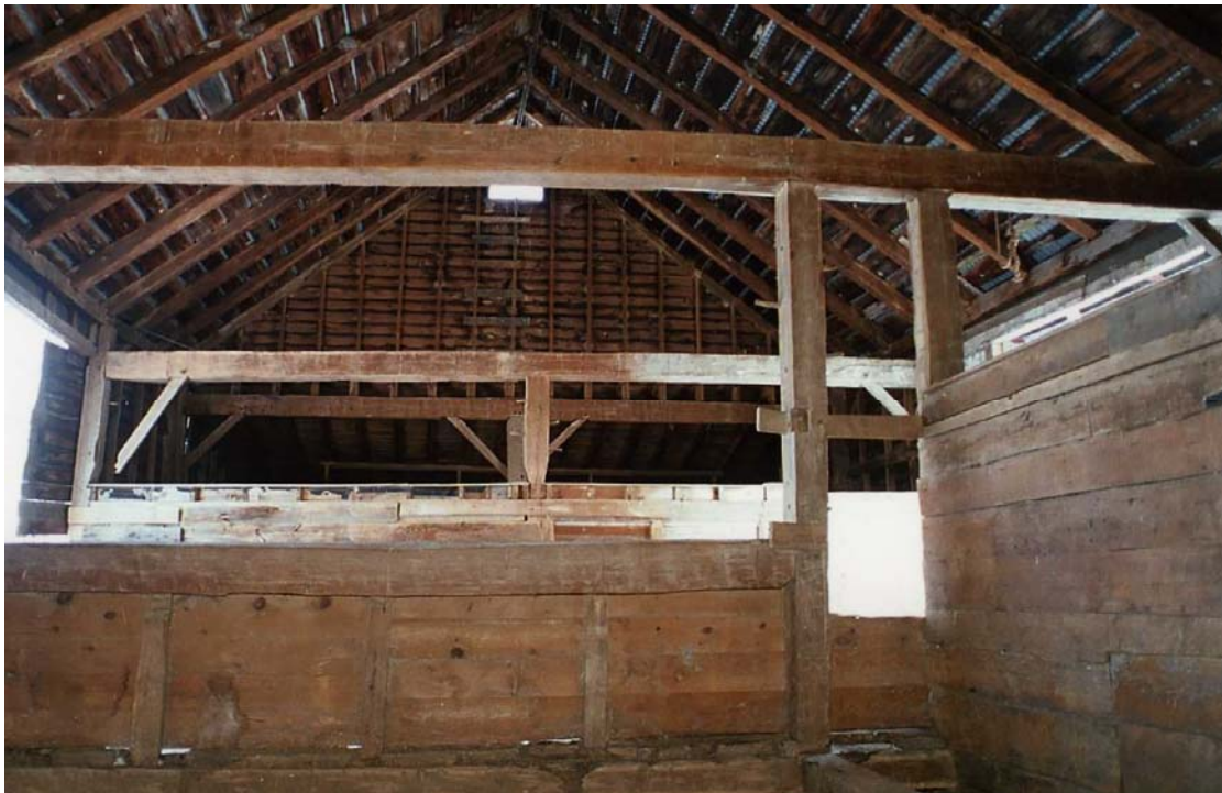
Figure 12. Interior of the Moseley barn, showing bents (photo by Connie Kheel, 2016).
