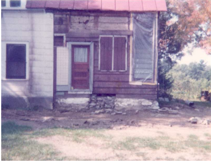
Figure 2 View of the Sharpe house after the removal of a small wing, exposing original shutters (Photograph by Sam Swanson, 1982).
